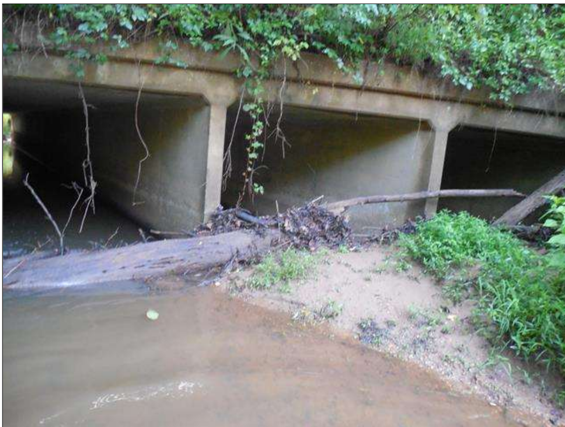
P.A.R. ISSUED FOR DRIFT AT INLET END OF ALL BARRELS IN A 21FT WIDE X 3FT HIGH X 2FT OUT AREA.
