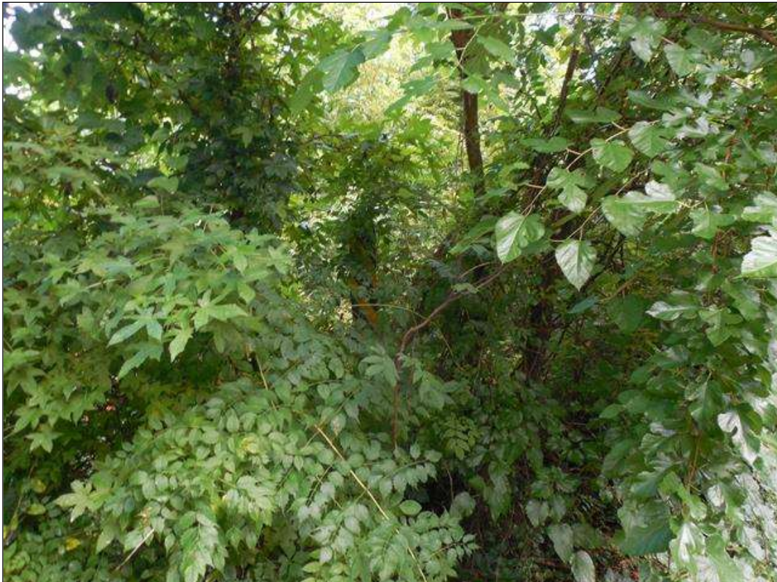
P.A.R. ISSUED FOR 1 MISSING DELINEATOR AT SOUTHWEST CORNER OF STRUCTURE. DELINEATOR IS BURRIED IN TREES AND VEGGIEITATION AND IS NOT VISIBLE FROM ROAD .
