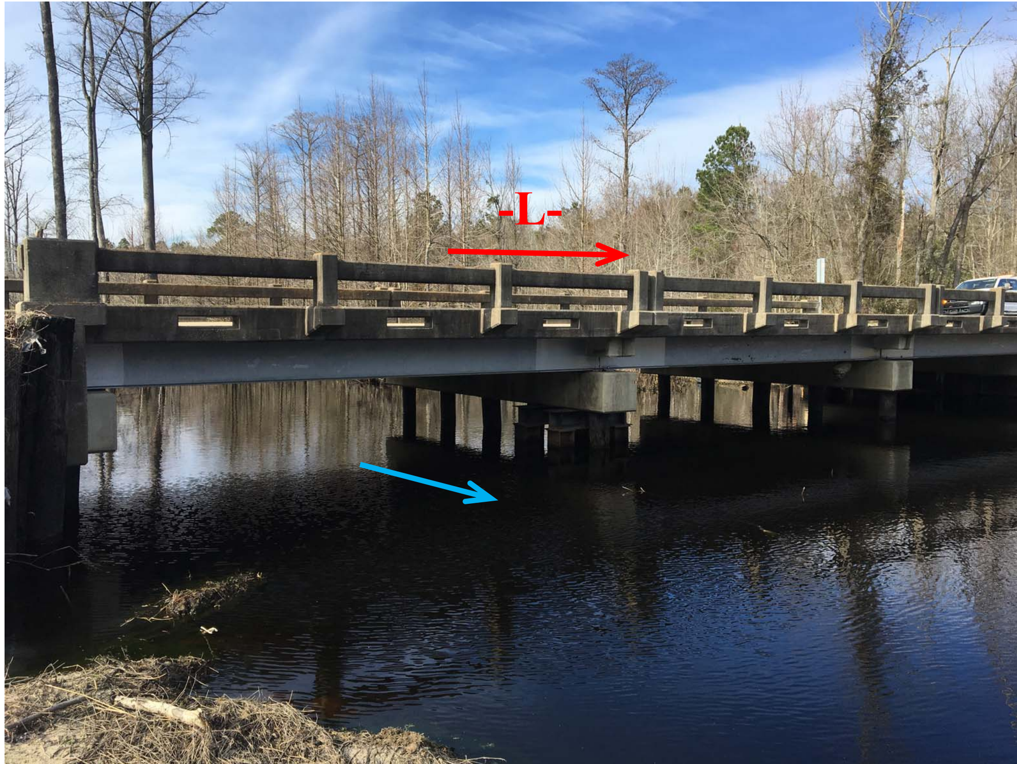
Looking Northeast towards End Bent 2
