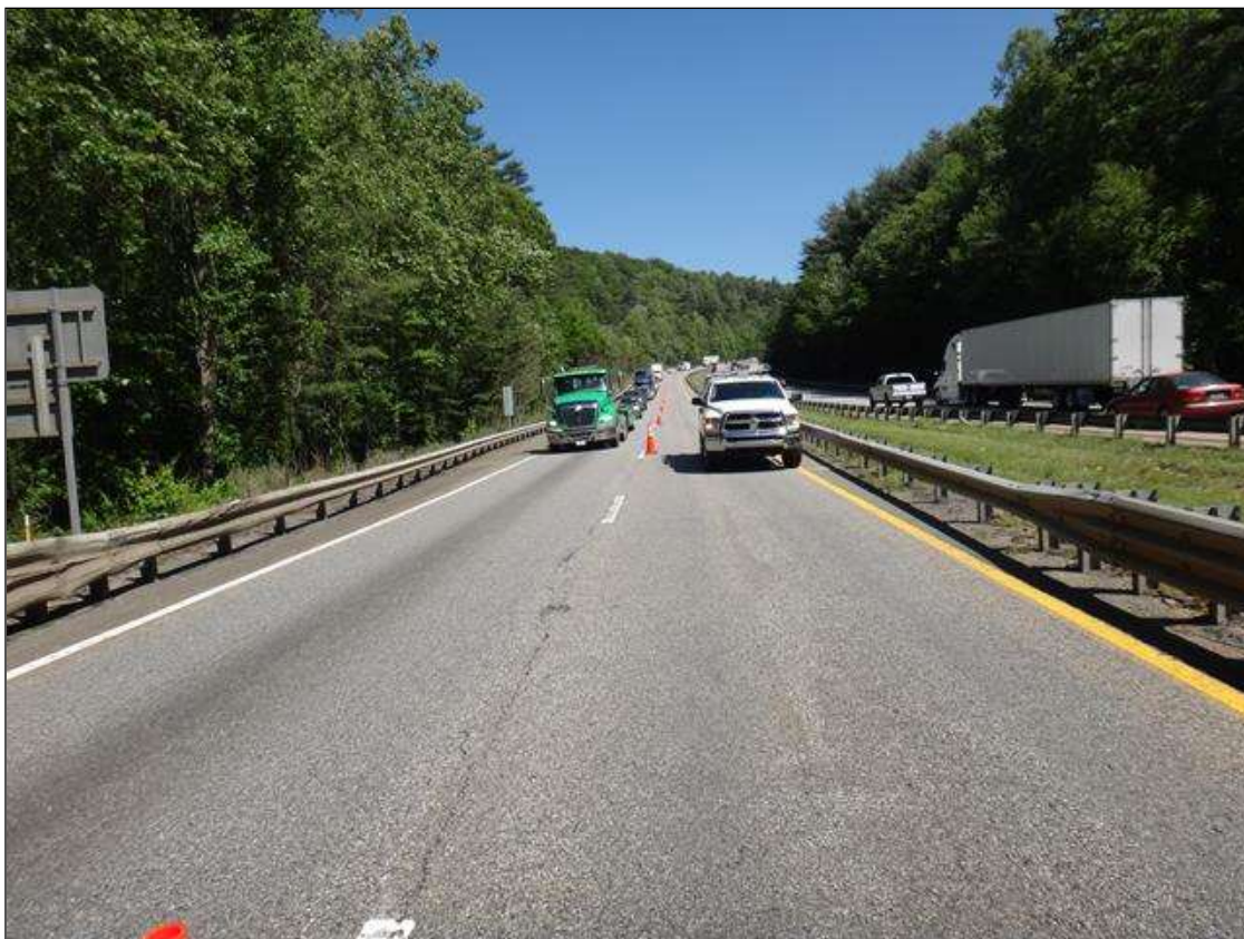
South approach looking South
