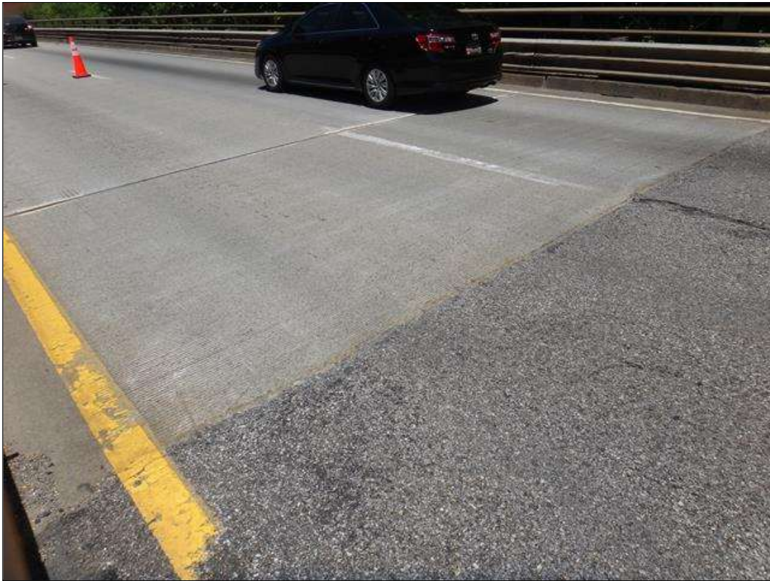
South approach asphalt
