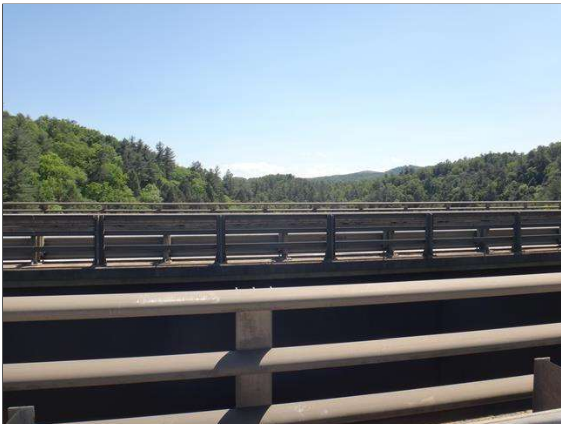
looking upstream [West] from bridge
