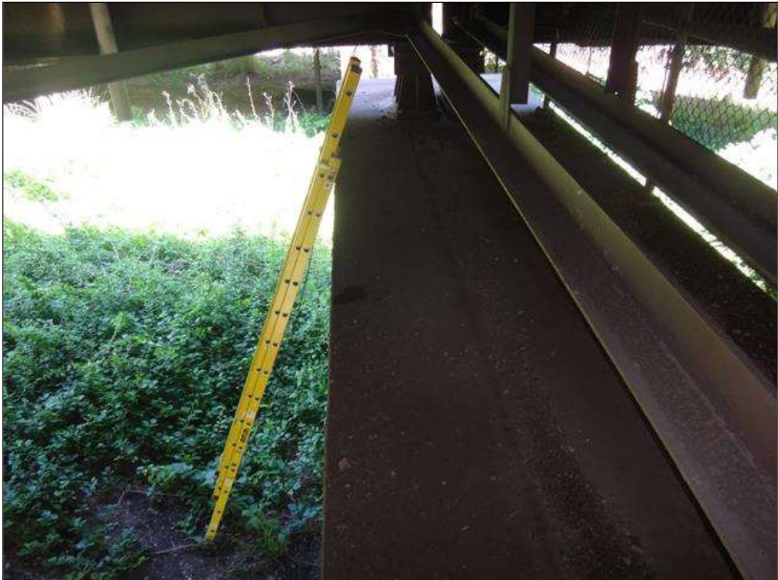
ladder access to bent 4 cap & catwalk
