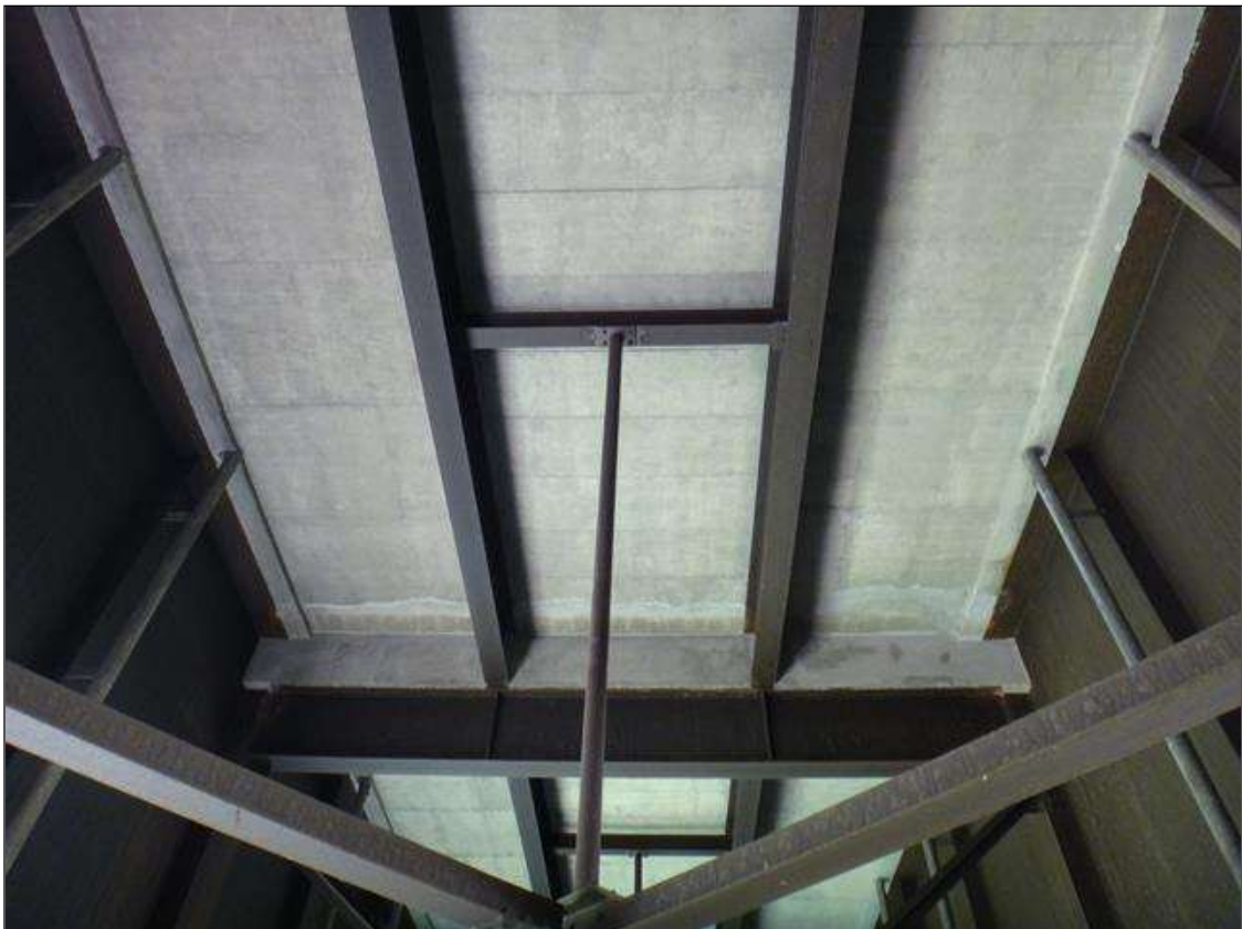
typical interior diaphragm
