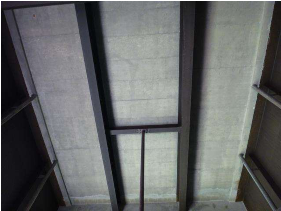
typical underside of deck
