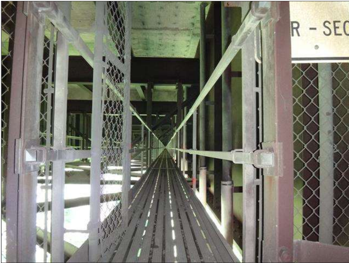
typical catwalk access
