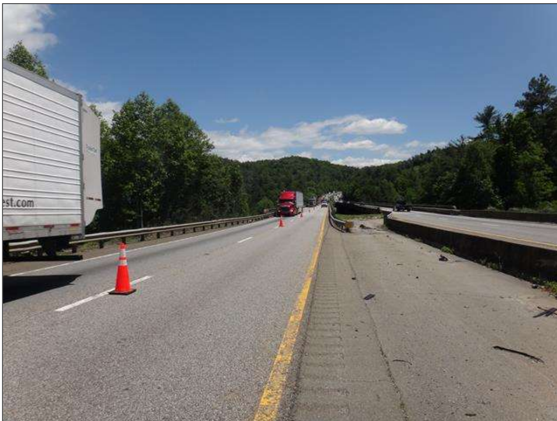
North approach looking South
