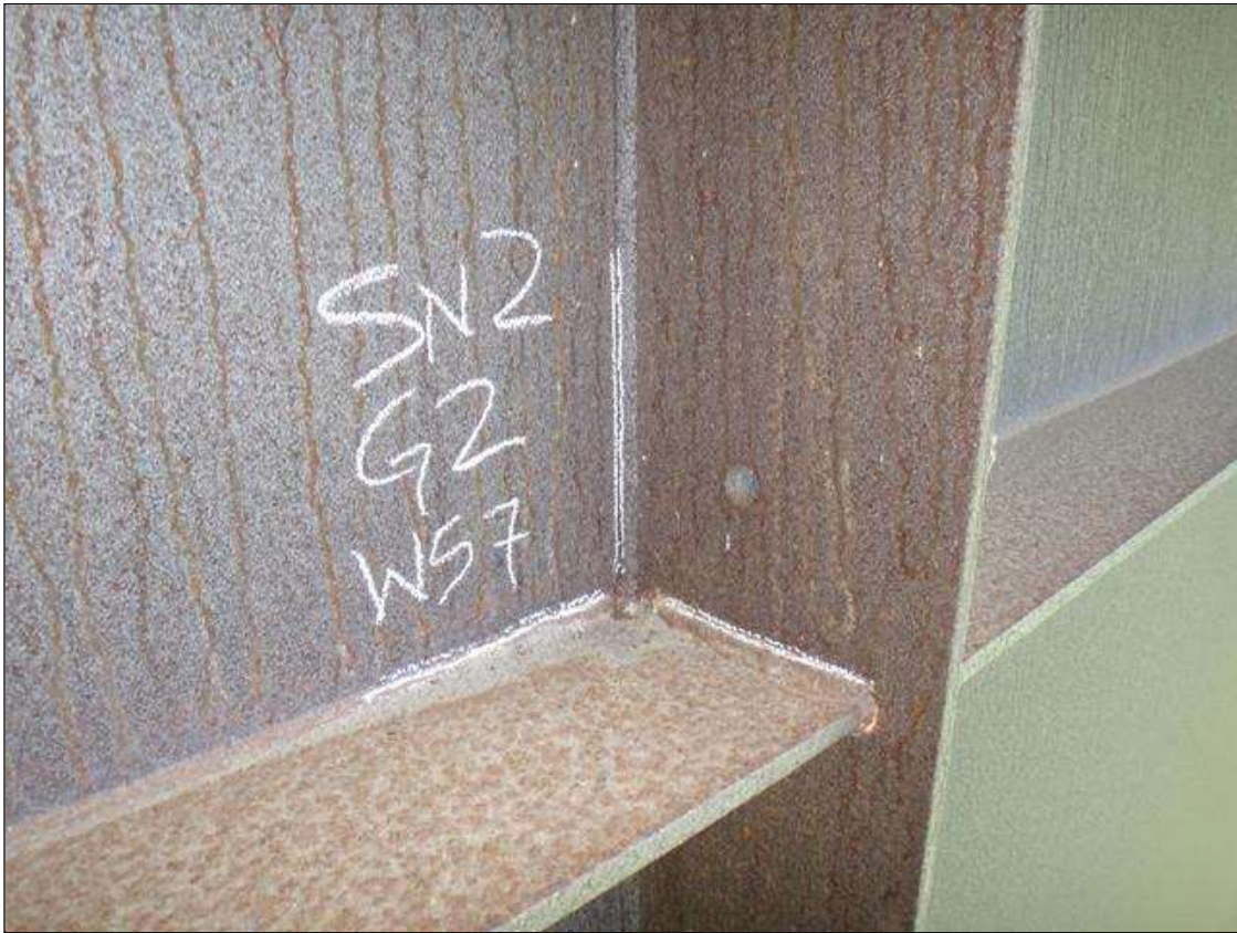
typical horizontal stiffener weld connection
