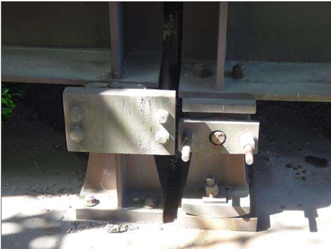
typical interior bearing [bent 1 & bent 4]
