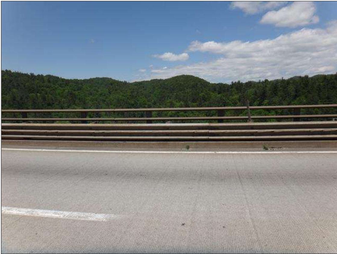
looking downstream [East] from bridge
