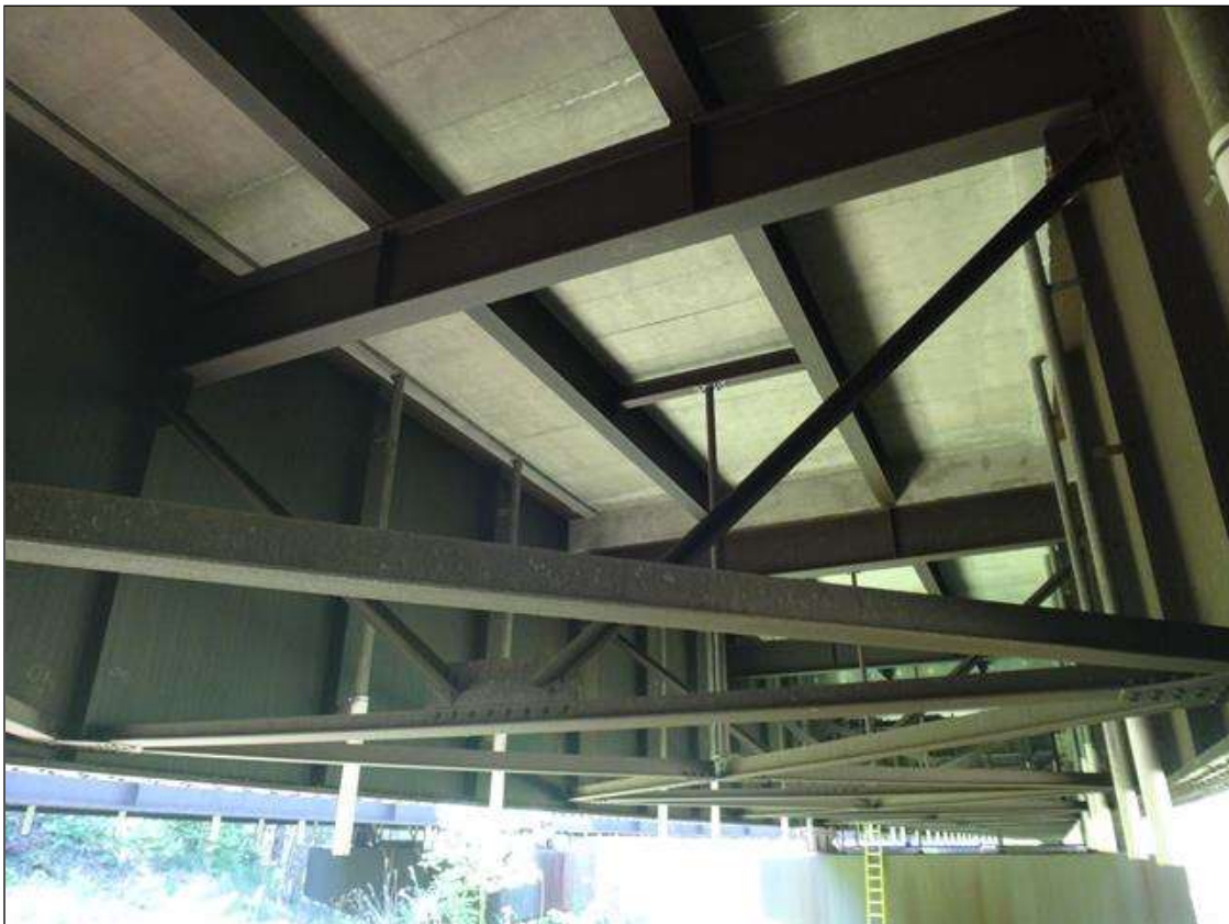
typical superstructure framing
