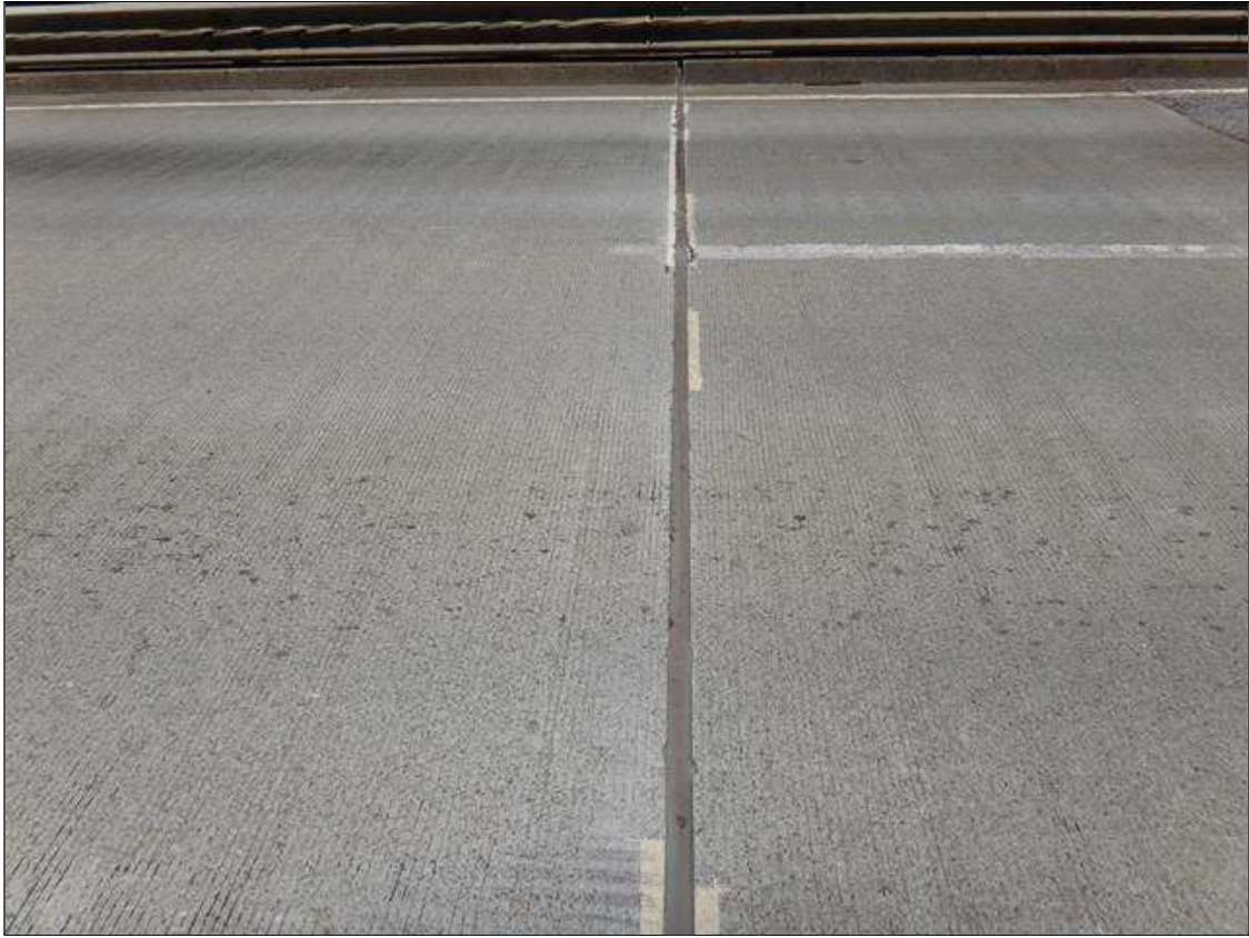
typical joint over end bent
