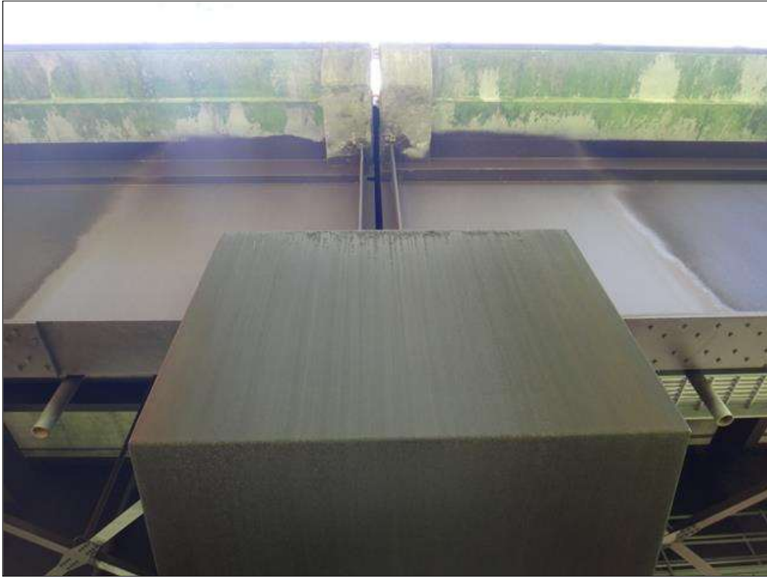
typical beam over interior bent
