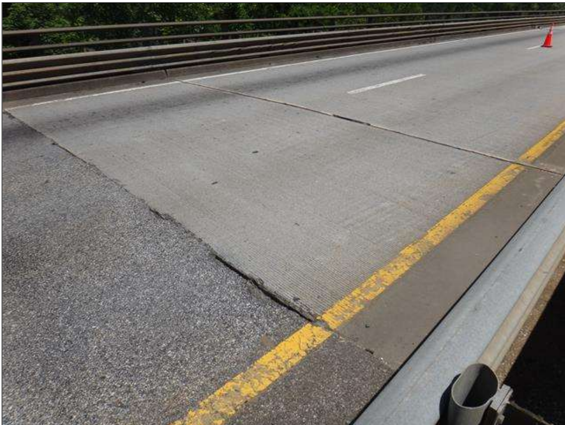
North approach asphalt
