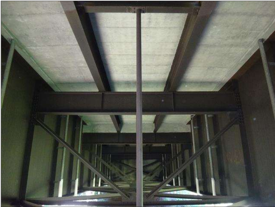
span 5 superstructure framing
