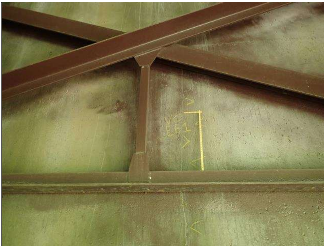
End Bent 1 Abutment/Backwall : at middle of backwall, vertical crack [full height x up to 0.02in]
