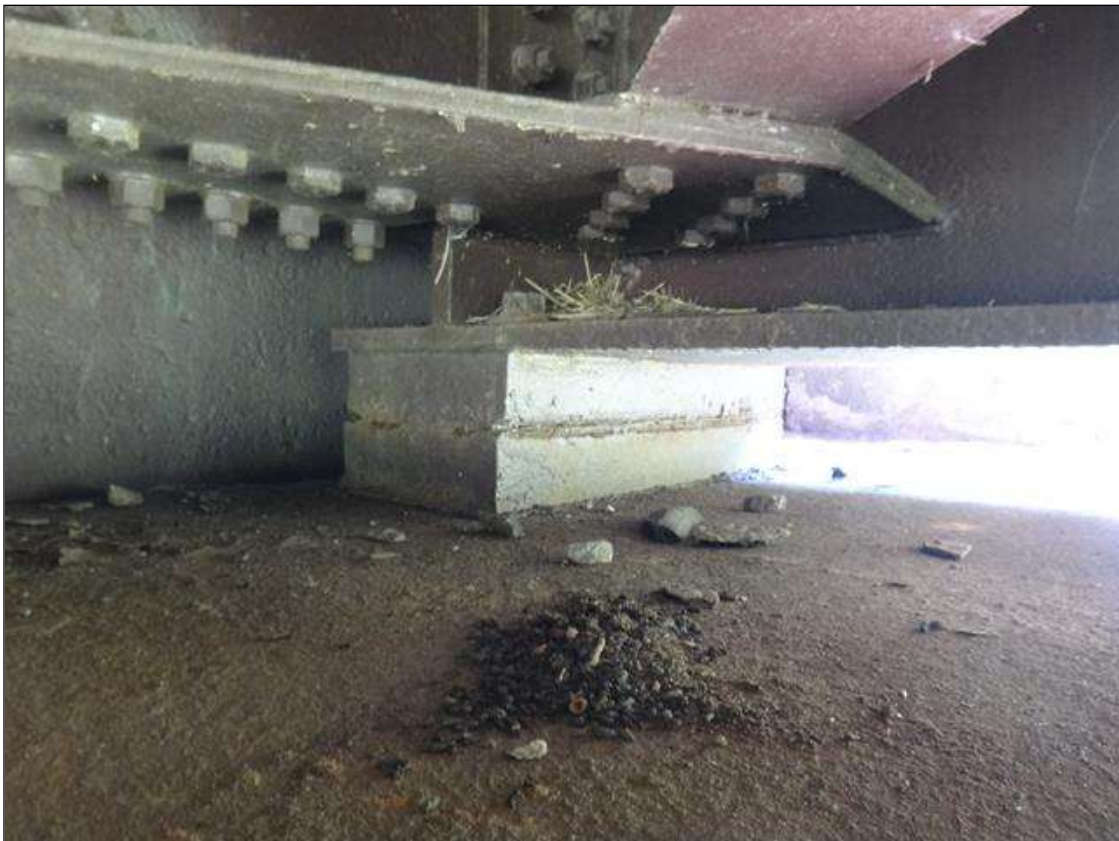
typical end bearing
