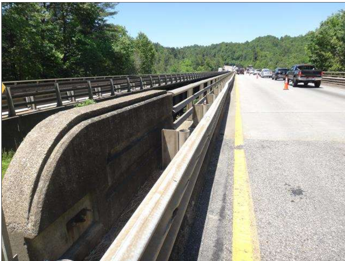
left bridge rail
