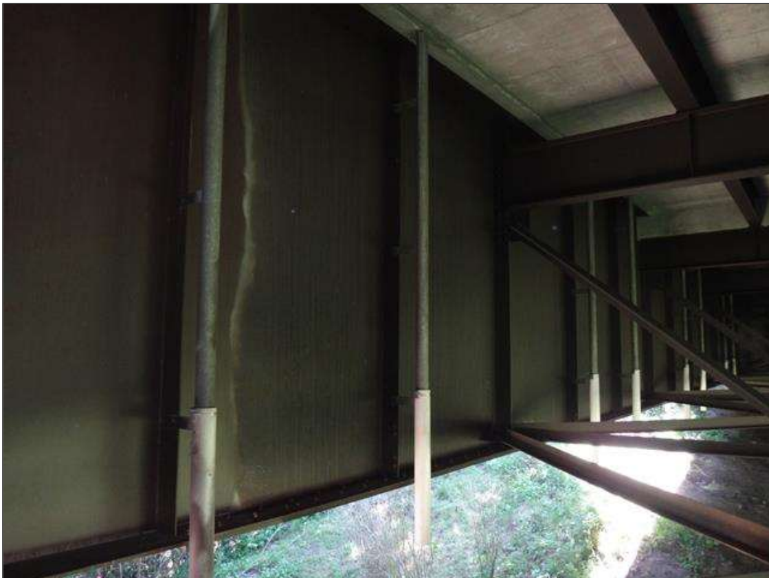
typical deck drain
