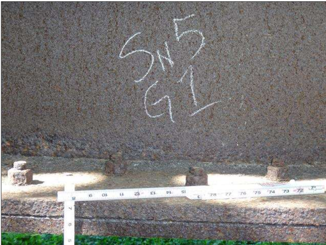
typical interior bearing
