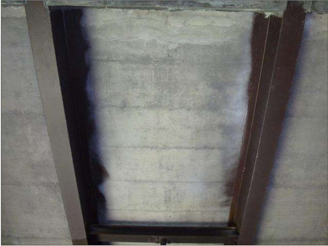
typical underside of deck
