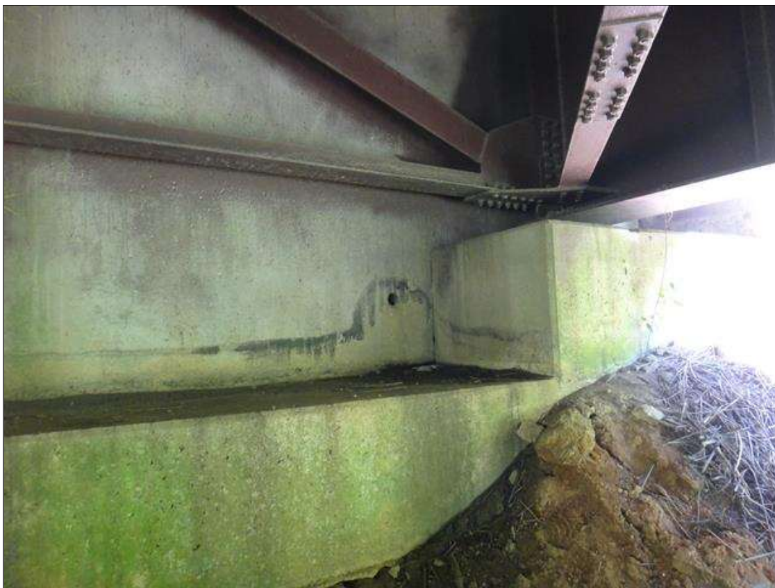
typical weep drain
