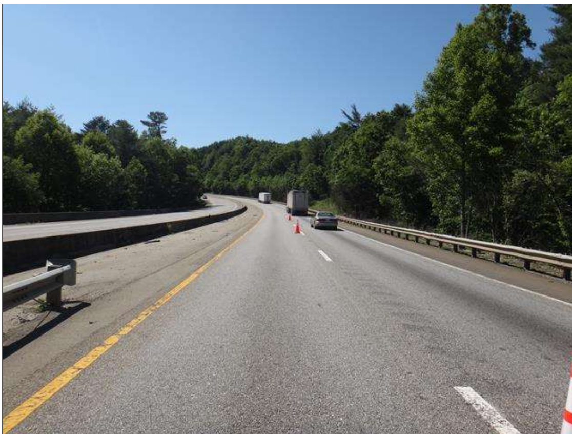
North approach looking North
