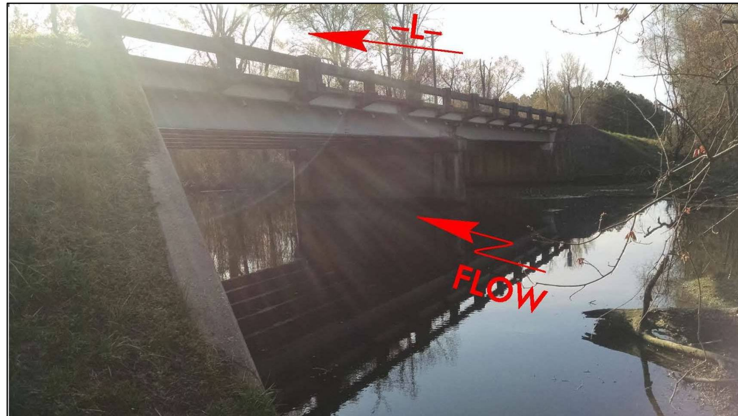
BRIDGE NO. 36 ON US 11 OVER MAXWELL CREEK
