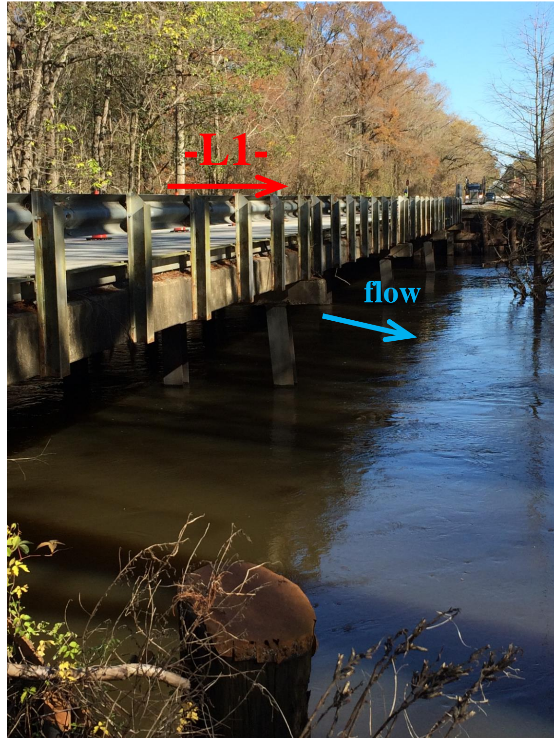
Looking North towards End Bent 2
