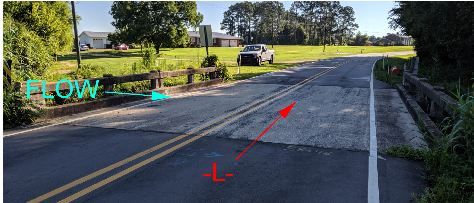
LOOKING EAST FROM END BENT 1 TOWARD END BENT 2
