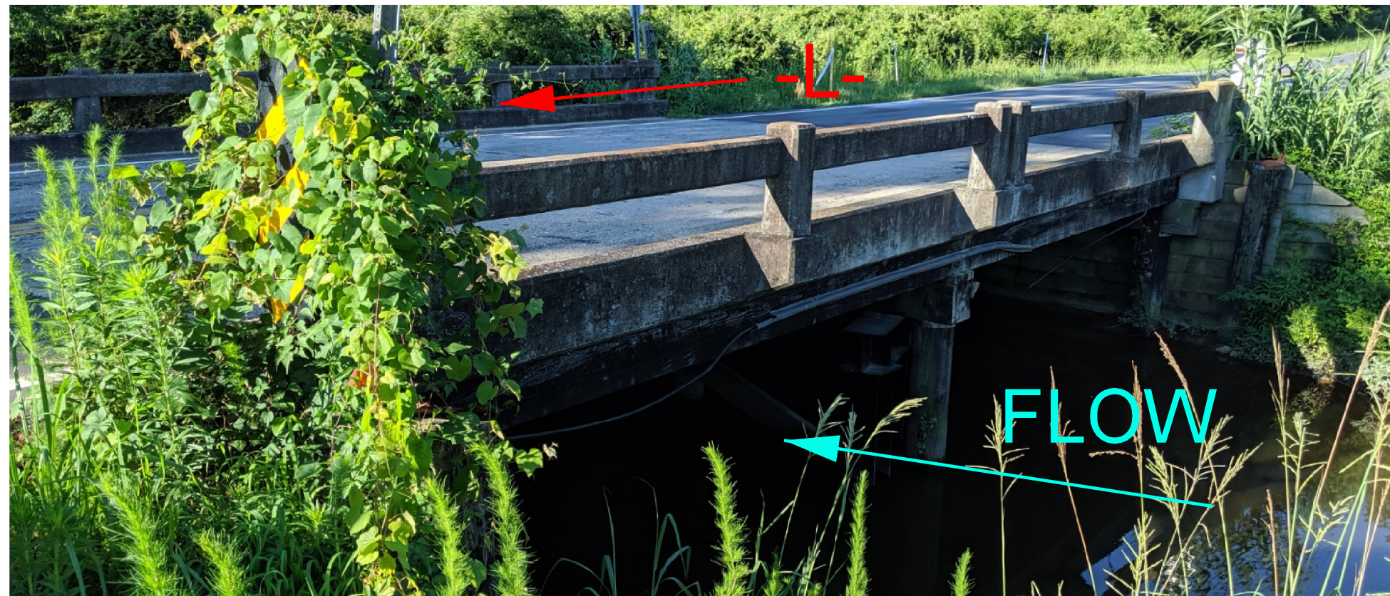
LOOKING SOUTH (DOWNSTREAM) TOWARD END BENT 1
