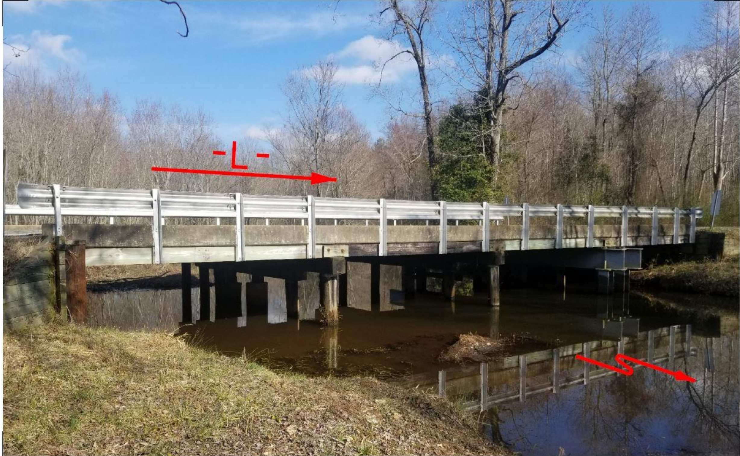
Looking East towards End Bent 2
