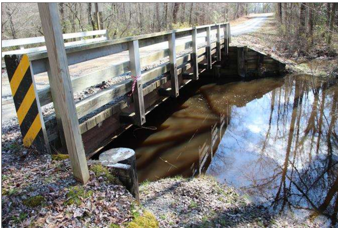
UPSTREAM/SOUTH PROFILE LOOKING EAST.
