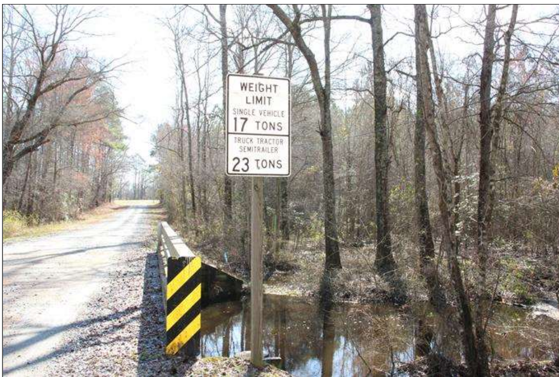
WEIGHT LIMIT SIGN AT SOUTHWEST CORNER.
