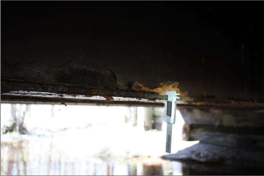
Span 1 Beam 5: HEAVY SURFACE CORROSION FOR FULL FLANGE WIDTH X 7 FT LONG IN BOTTOM FLANGE, STARTING AT 13.5 FT FROM BEAM END AT END BENT 1 . UP TO 0.41 IN SECTION REMANING (PAR).
