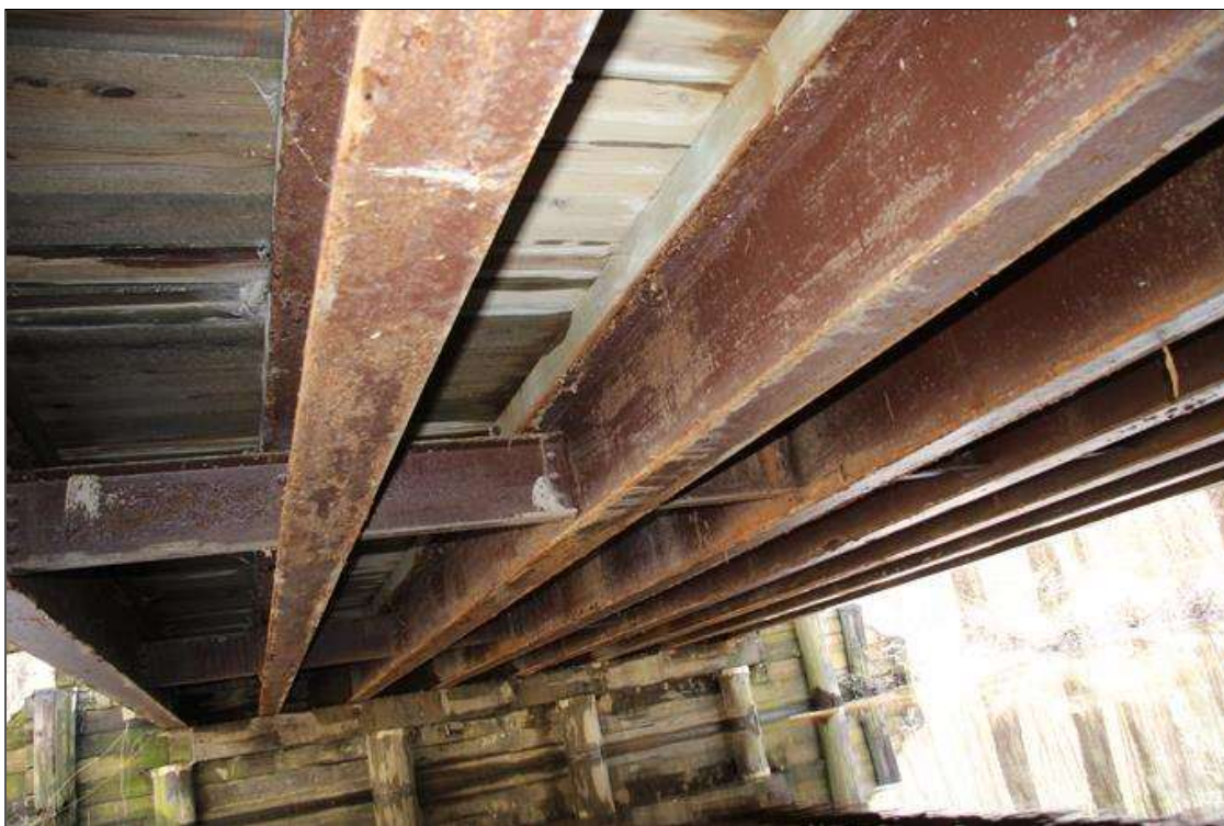
SUPERSTRUCTURE UNDERSIDE LOOKING EAST.
