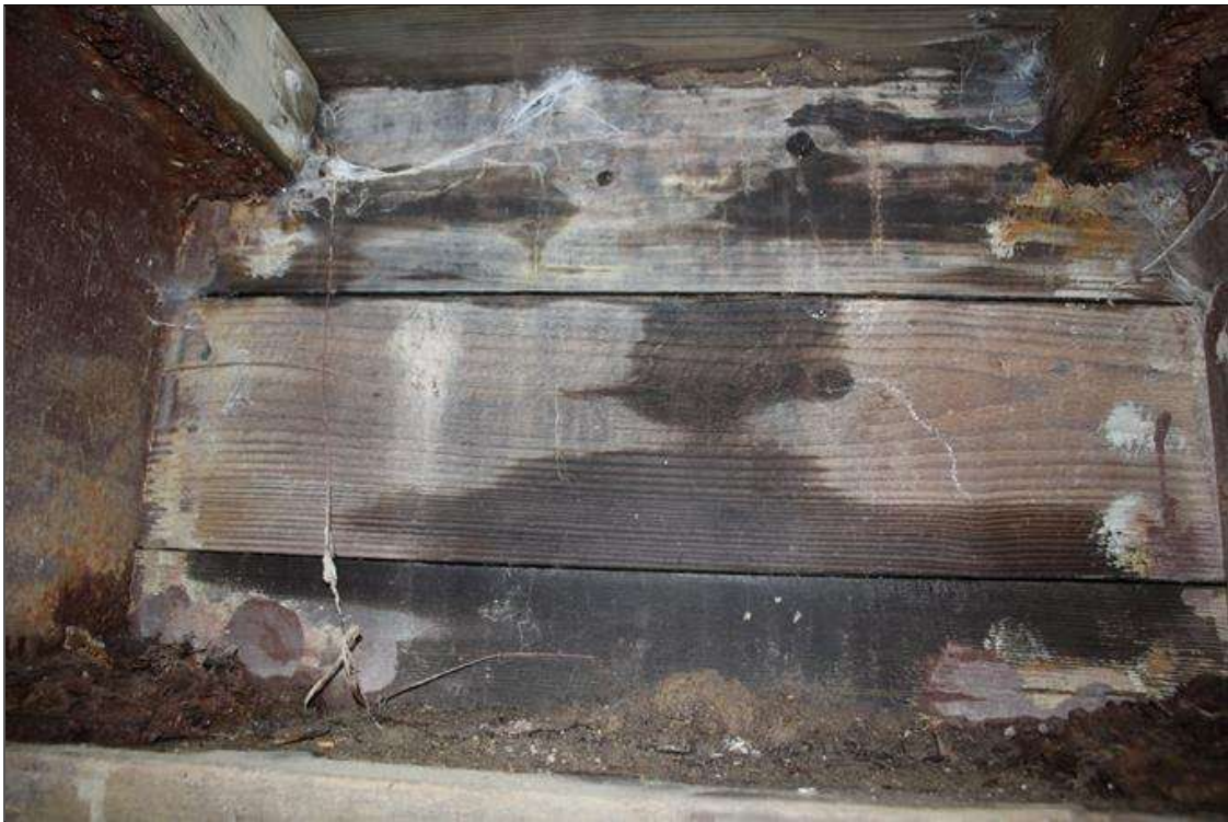
BACKWALL AT END BENT 1, BAY 1.
