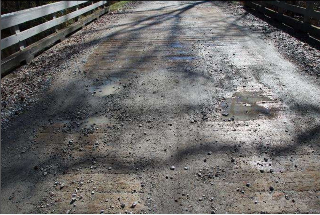
TOP OF DECK LOOKING EAST.
