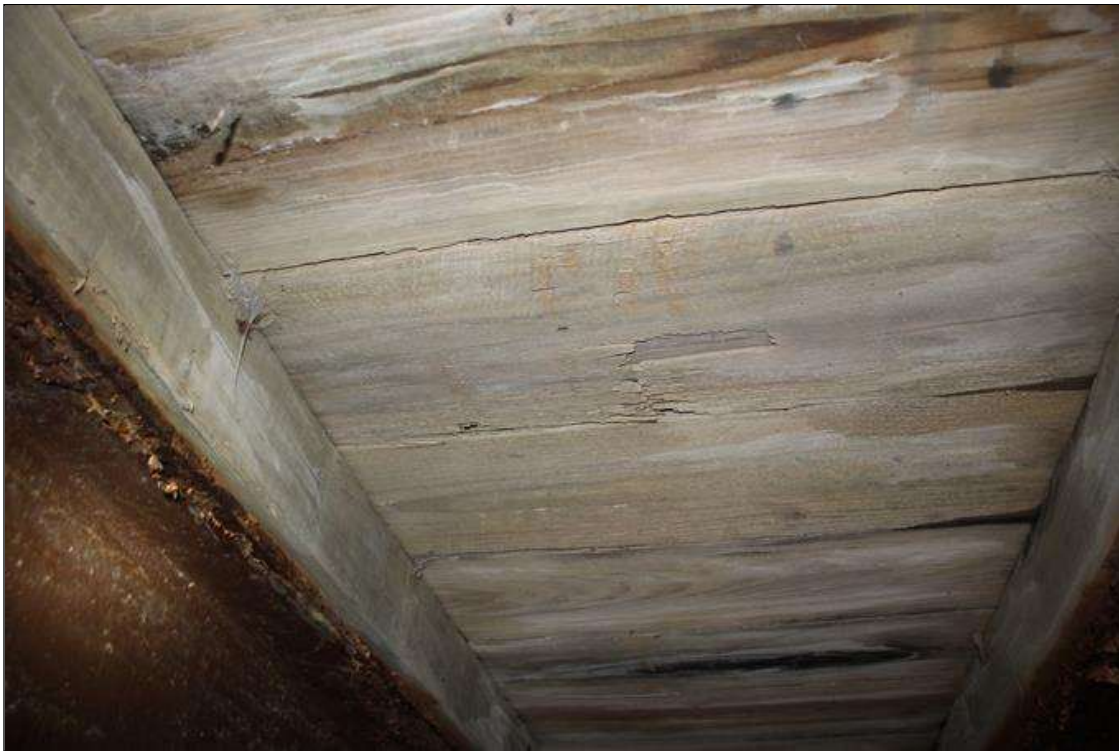
TYPICAL DECK UNDERSIDE IN BAY 4 AT END BENT 1, LOOKING WEST.
