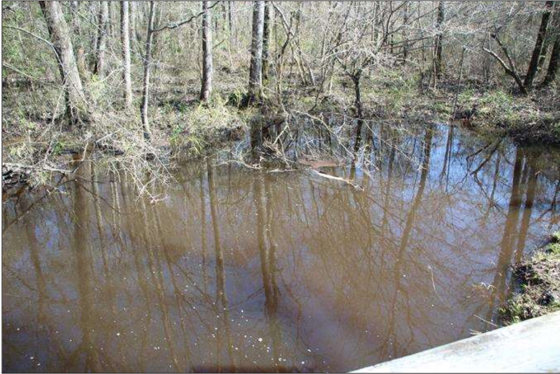
DOWNSTREAM LOOKING NORTH FROM TOP OF DECK.
