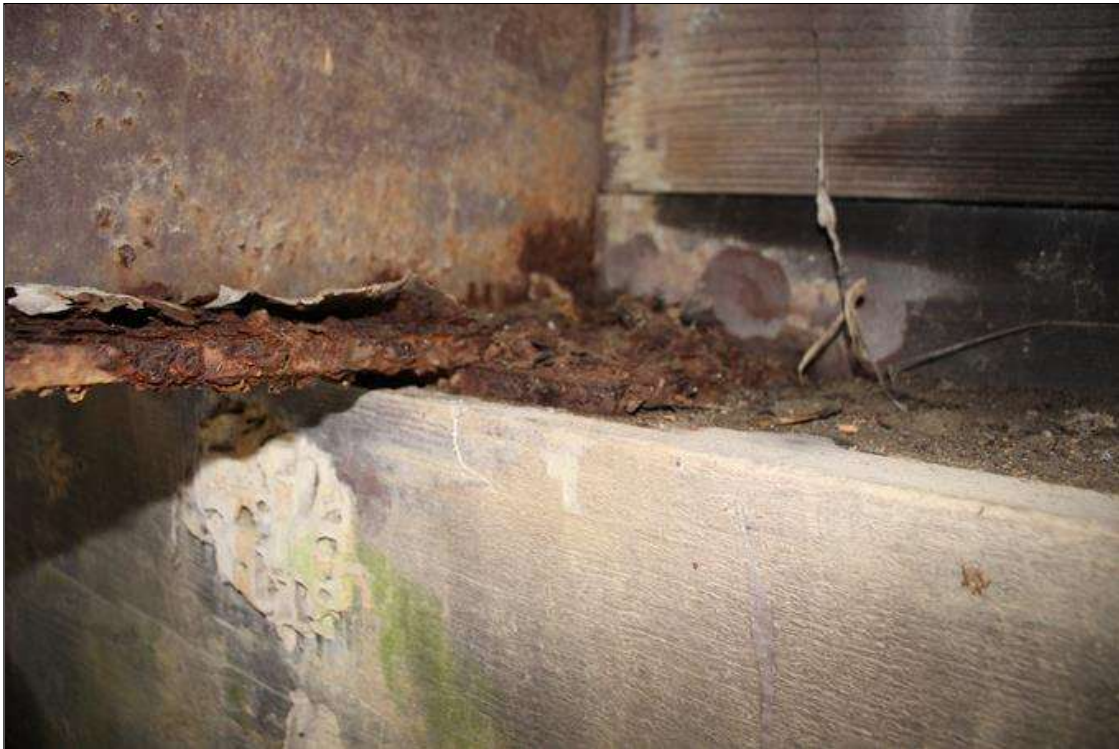
BEARING AT END BENT 1 BEAM 2.
