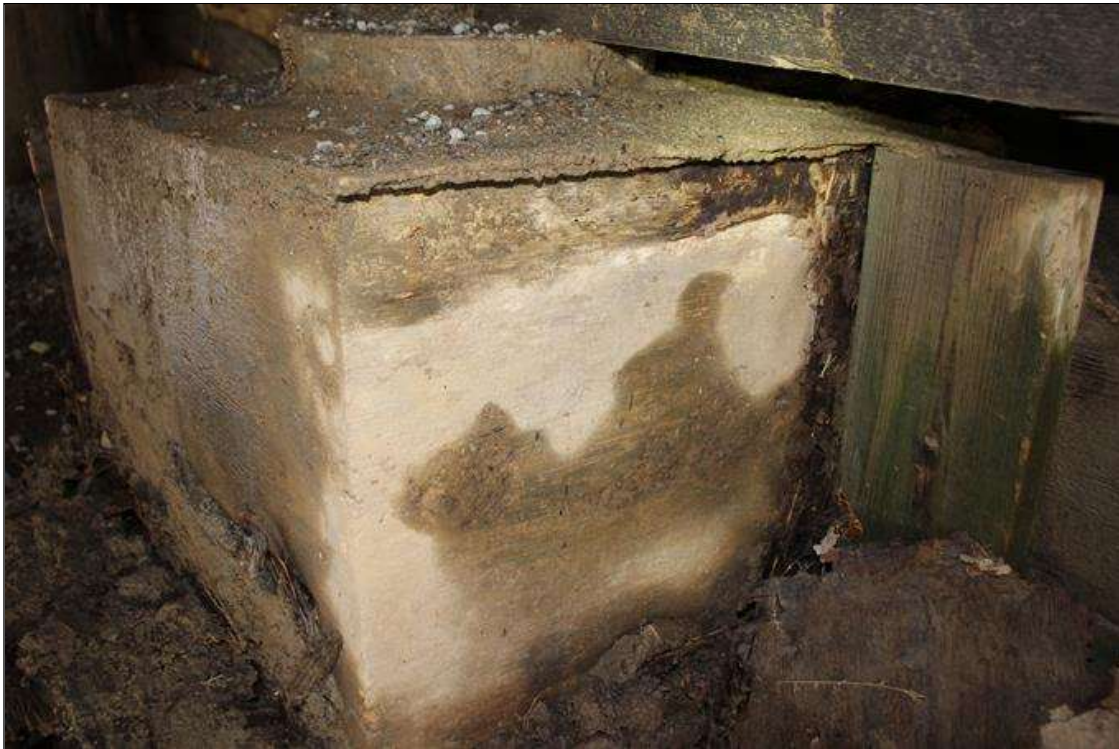
PILE 2 AT END BENT 1 IS ENCASED IN CONCRETE.
