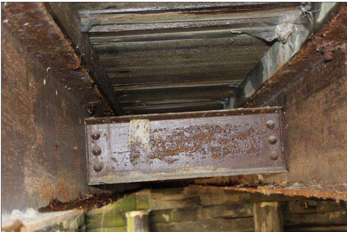
INTERMEDIATE DIAPHRAGM IN BAY 1 LOOKING EAST.
