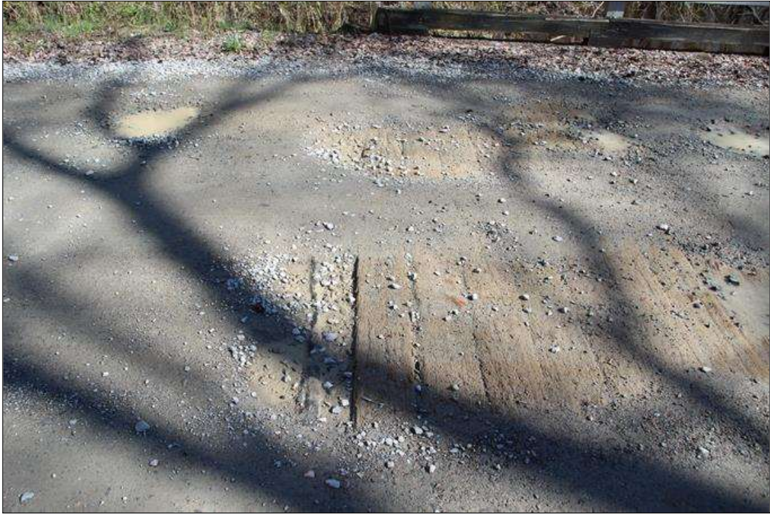
DECK OVER END BENT 1 LOOKING NORTH. SIMILAR AT END BENT 2.
