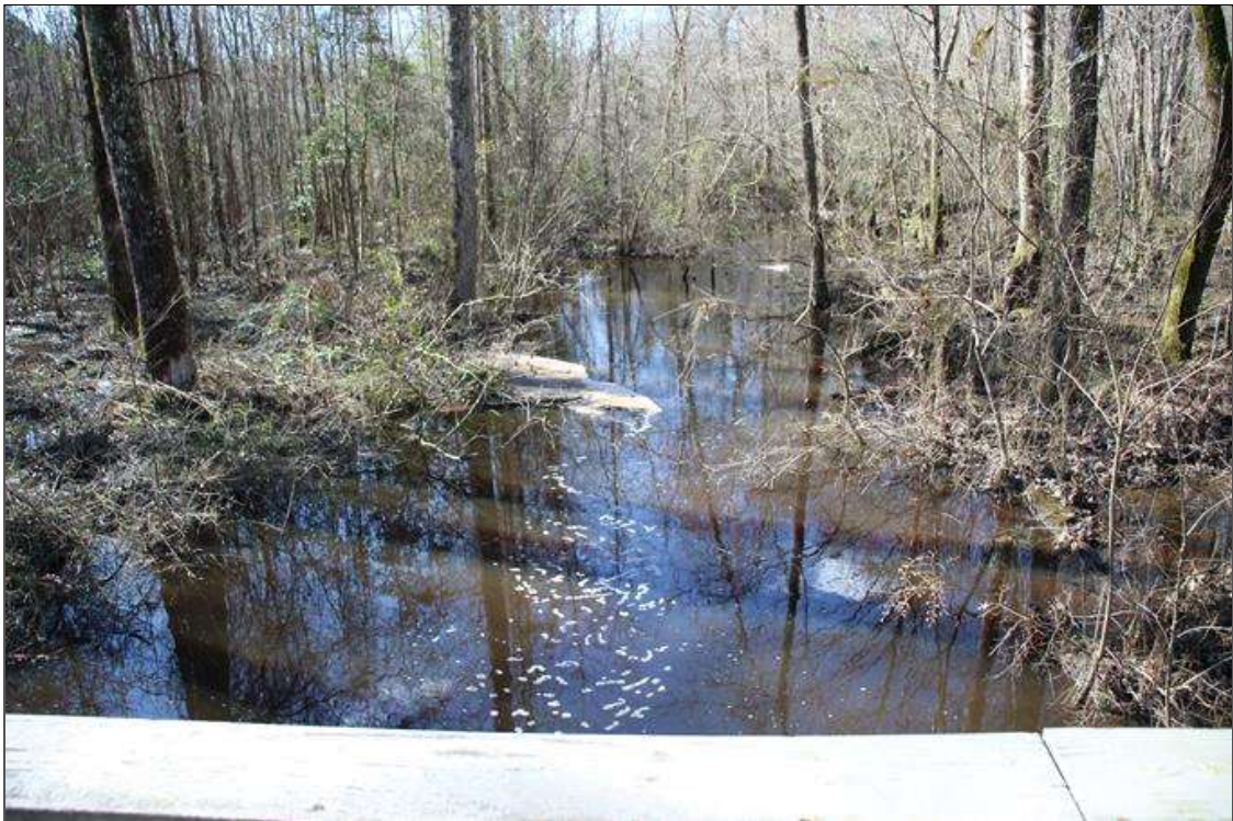
UPSTREAM LOOKING SOUTH FROM TOP OF DECK.
