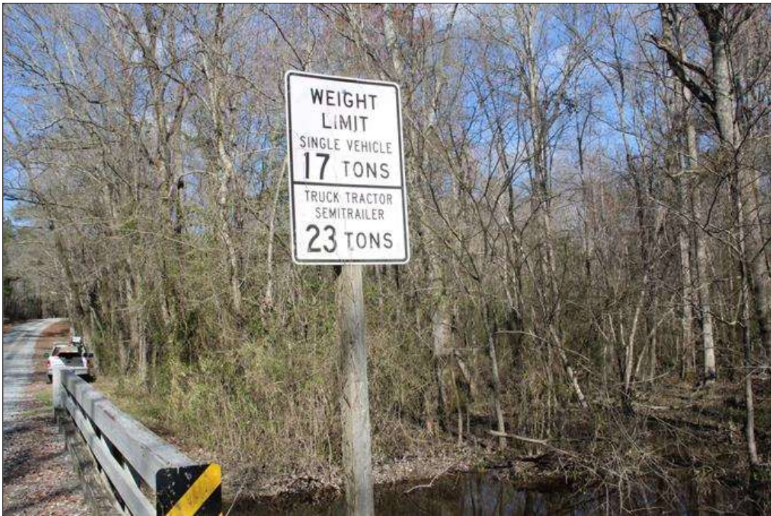
WEIGHT LIMIT SIGN AT NORTHEAST CORNER.
