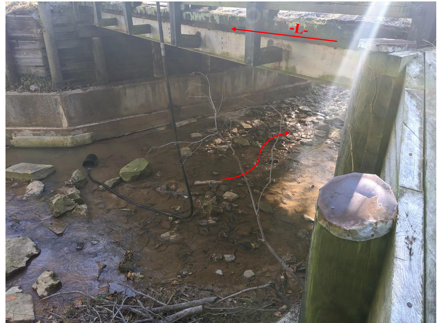
Photograph No. 2: Looking Upstream
