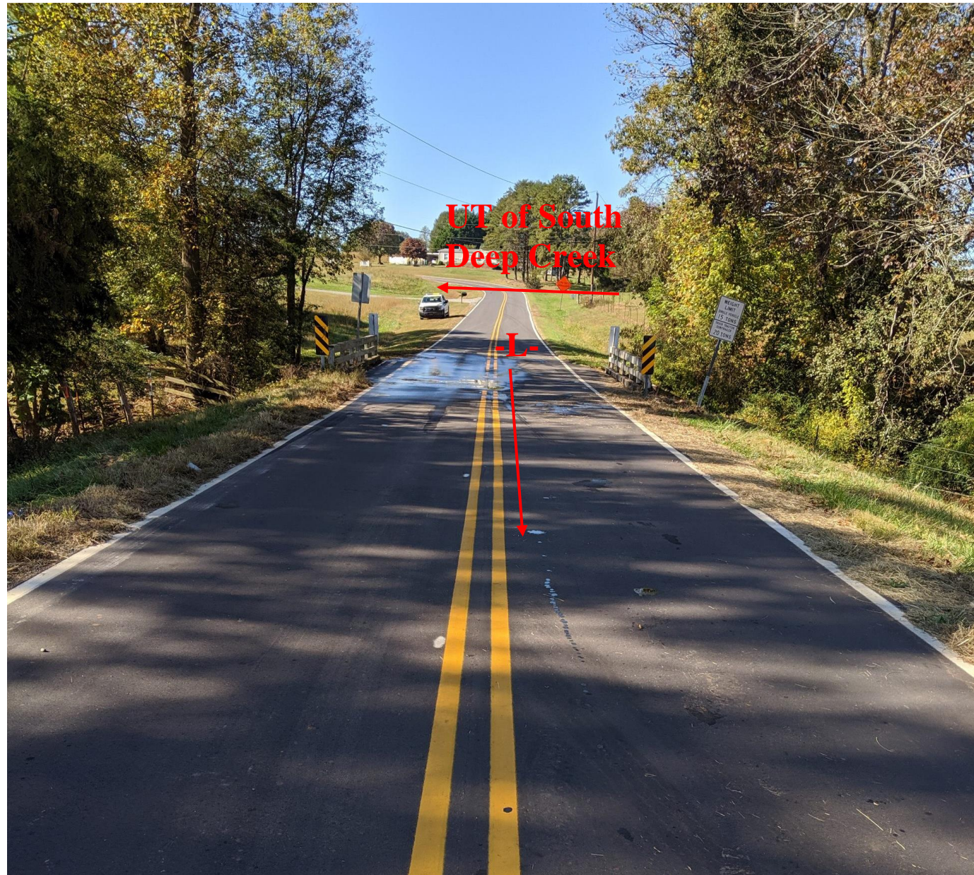
Photograph No. 1: Looking at End Bent 2 toward End Bent 1
