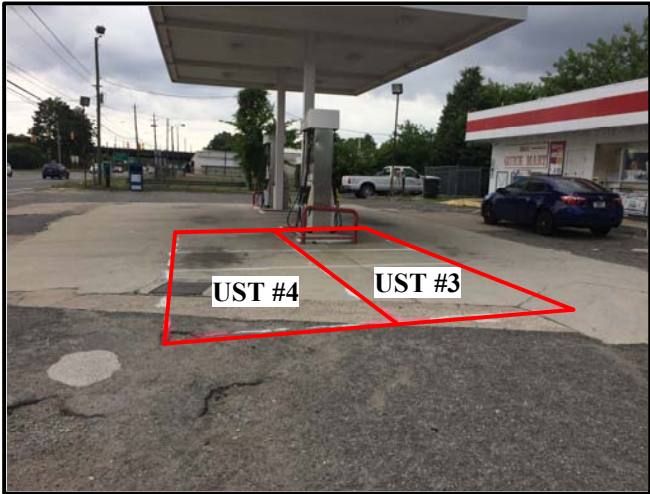
View of Probable UST #3 & #4 Facing Approximately Southwest
