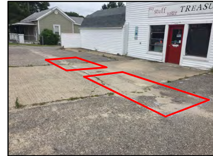
PROBABLE USTs #1 & #2 (FACING APPROXIMATELY NORTHEAST)
