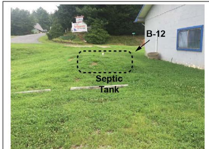
5. Septic tank for former auto repair facility and location of Boring B-13.
