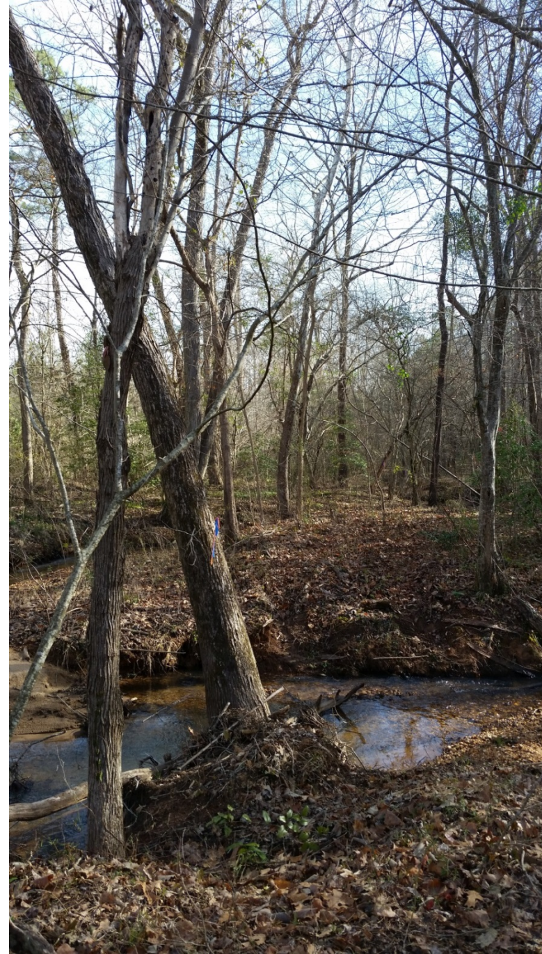
Photo 1: Looking East along Loop C Culvert
