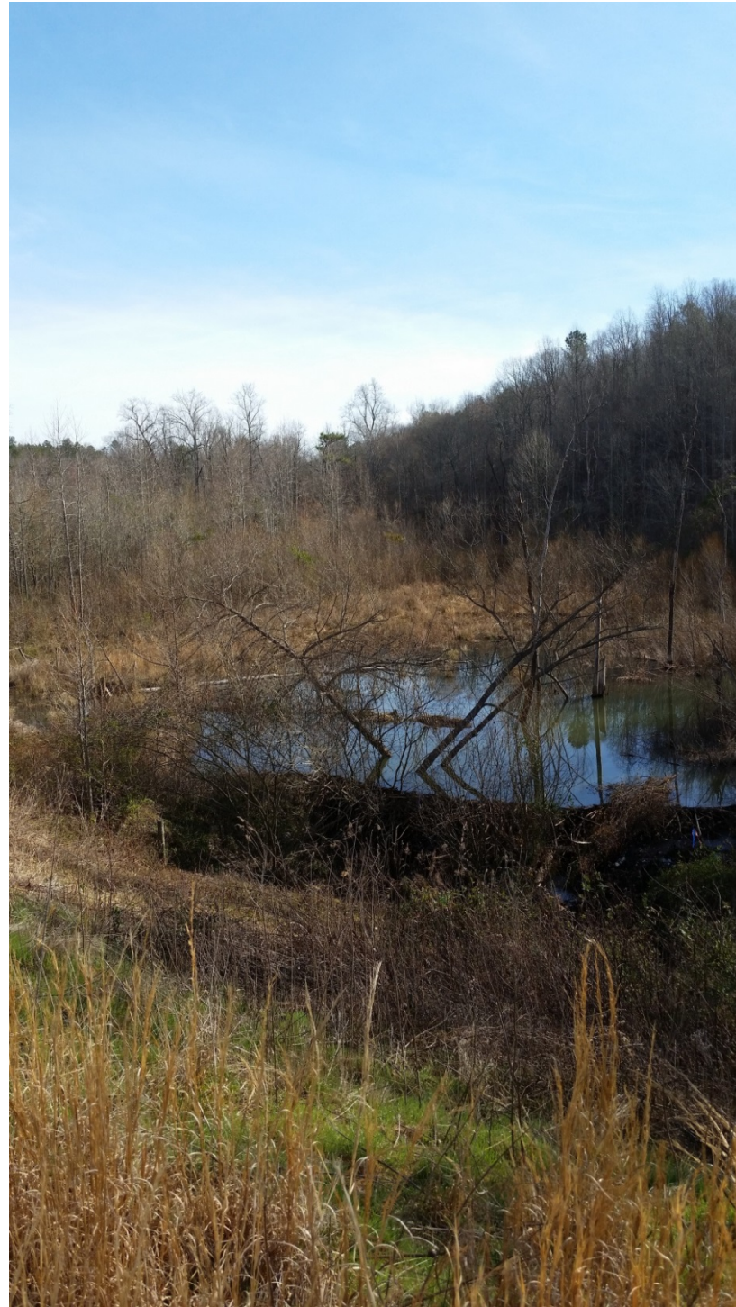
Photo 1: Looking East along the I73 Culvert
