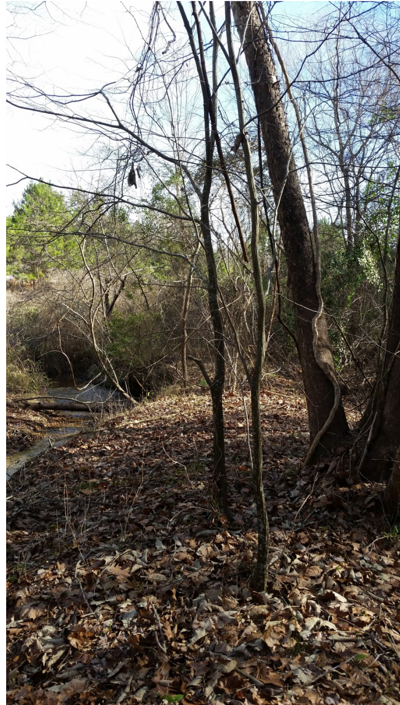
Photo 1: Looking North along Ramp C Culvert
