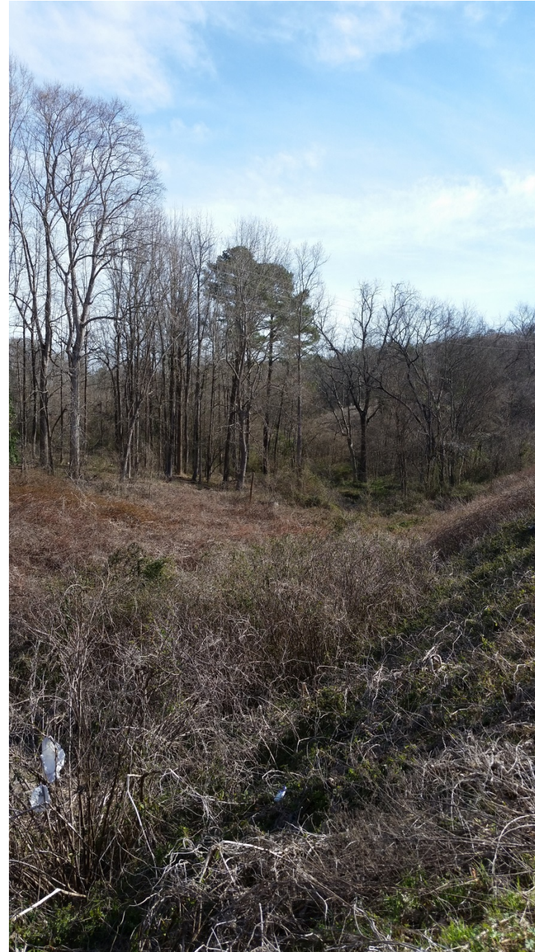
Photo 2: Looking North along Ramp C Culvert
