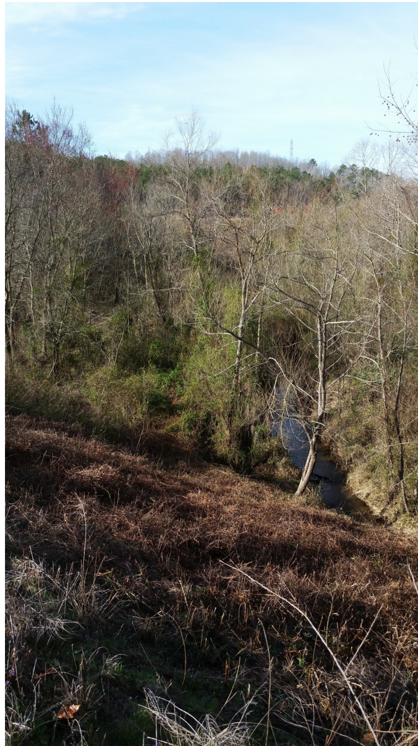
Photo 1: Looking South Along Loop B Culvert
