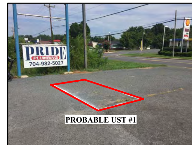
View of Probable UST #1 Facing Approximately Northwest
