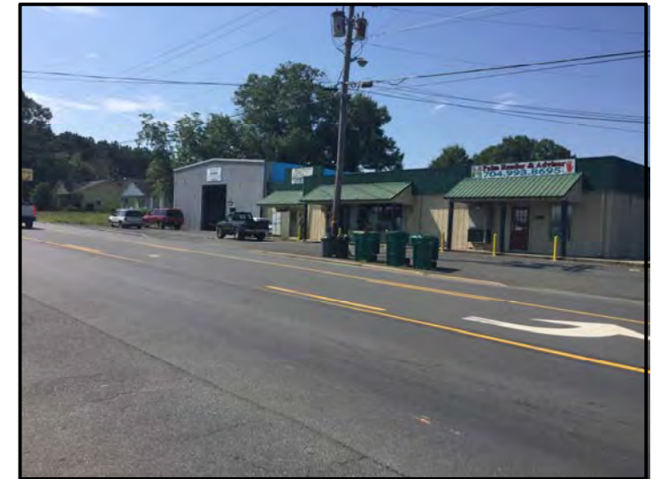
View of Survey Area (Facing Approximately Southeast)
