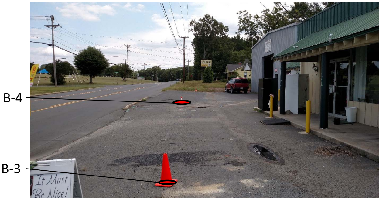
Photo #3: Boring locations B-3 and B-4, facing southeast.
