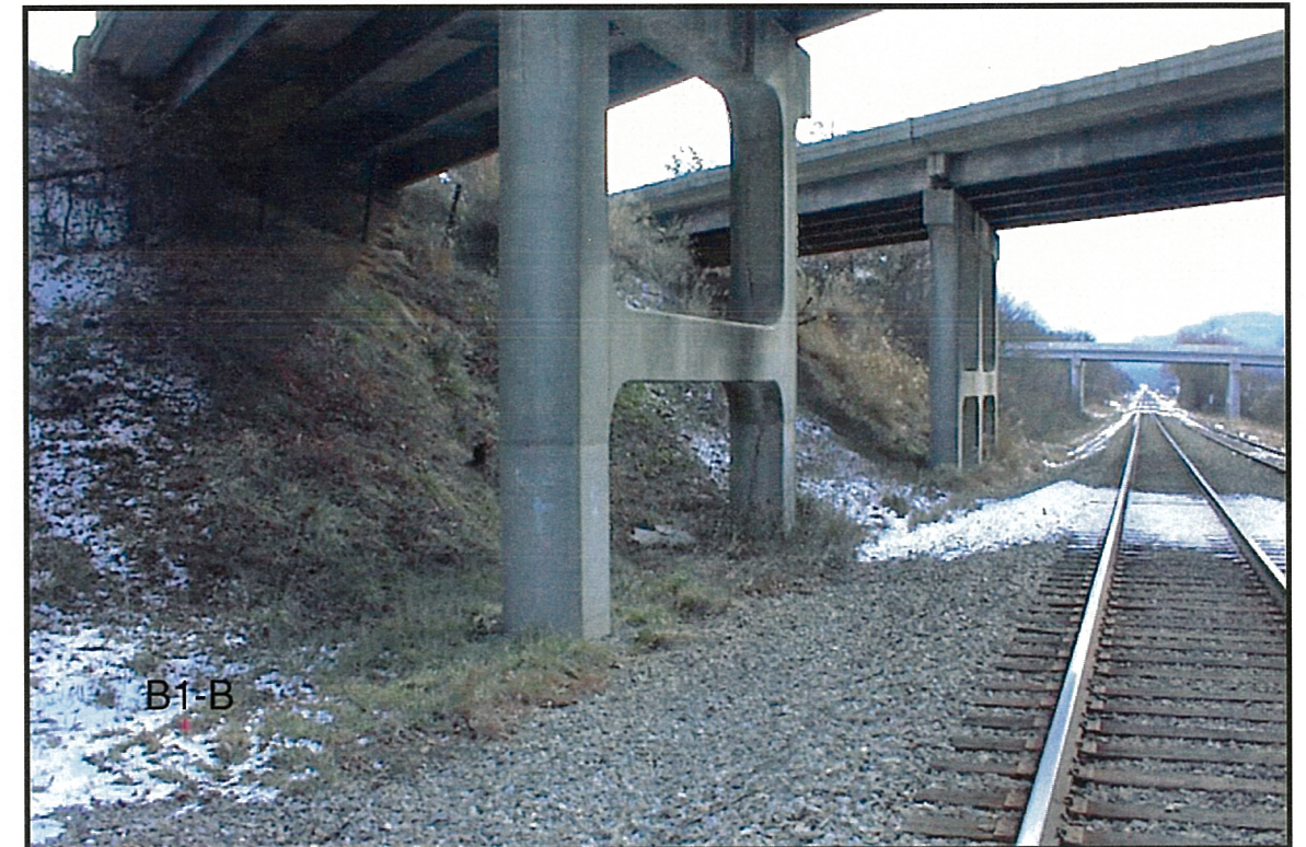
Photograph 4: View looking south along Bent 1. B1-B in foreground.
