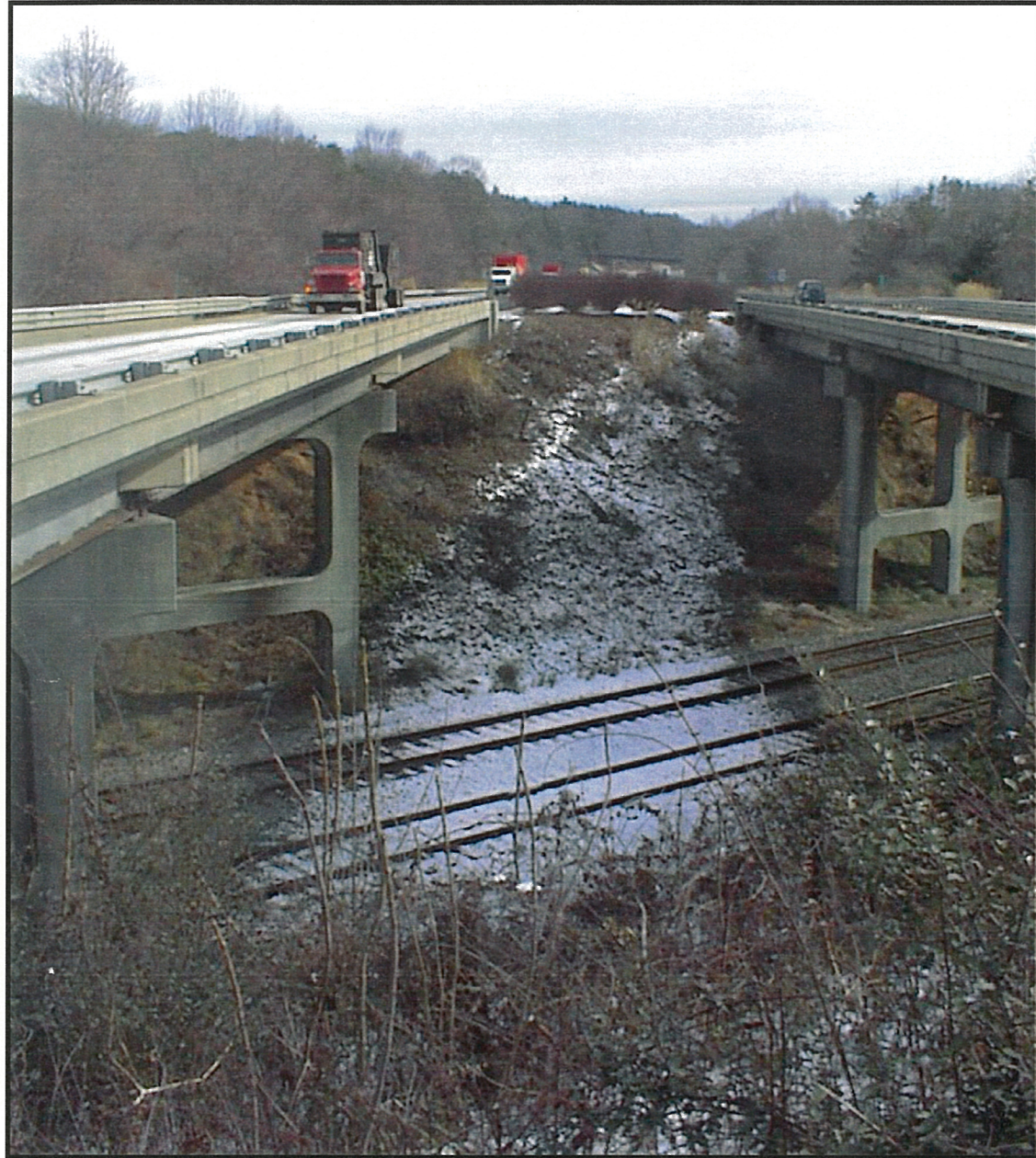
Photograph 9: View looking southeast along -L- toward End Bent 1.
