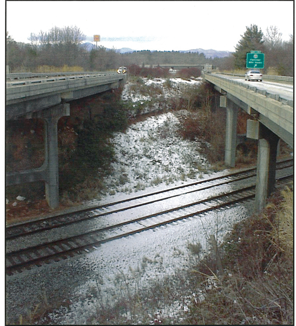
Photograph 10: View looking northwest along -L- toward End Bent 2.
