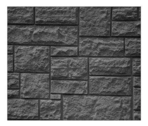
All texture is to be in addition to the nominal thickness of each element within tolerances. Maximum relief of the textured surface shall be 1¼ inch or less.
