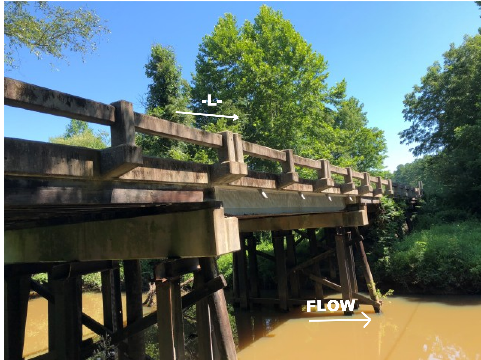
PHOTOGRAPH NO.1.: VIEW LOOKING NORTH.
