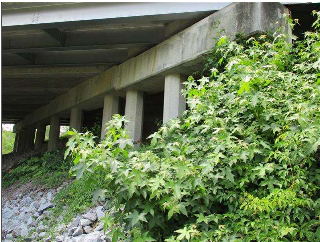
BENT 4 LOOKING NORTH
