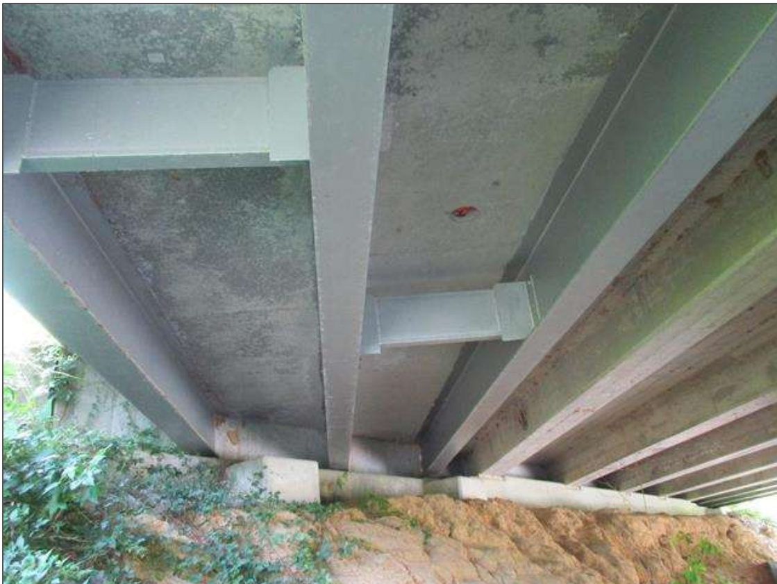
END BENT 1 LOOKING SOUTH
