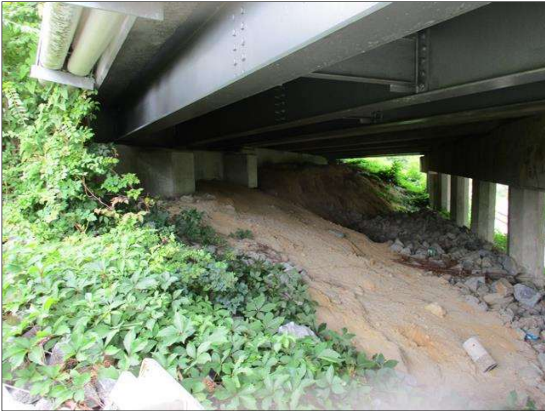
END BENT 2 LOOKING NORTH
