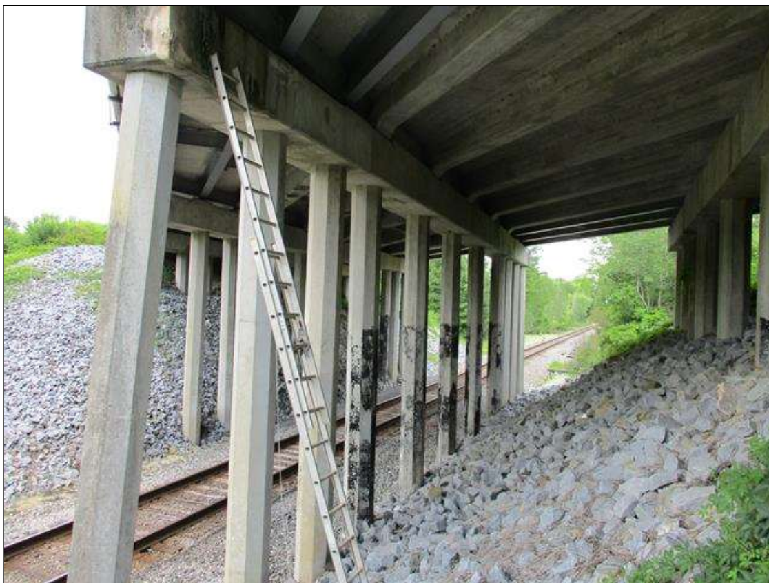
BENT 2 LOOKING NORTH
