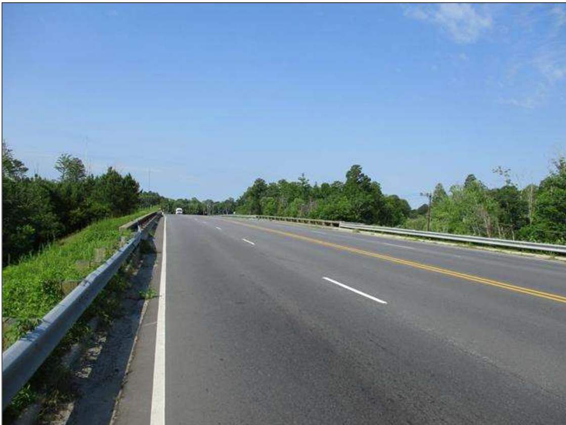
NORTH APPROACH LOOKING SOUTH
