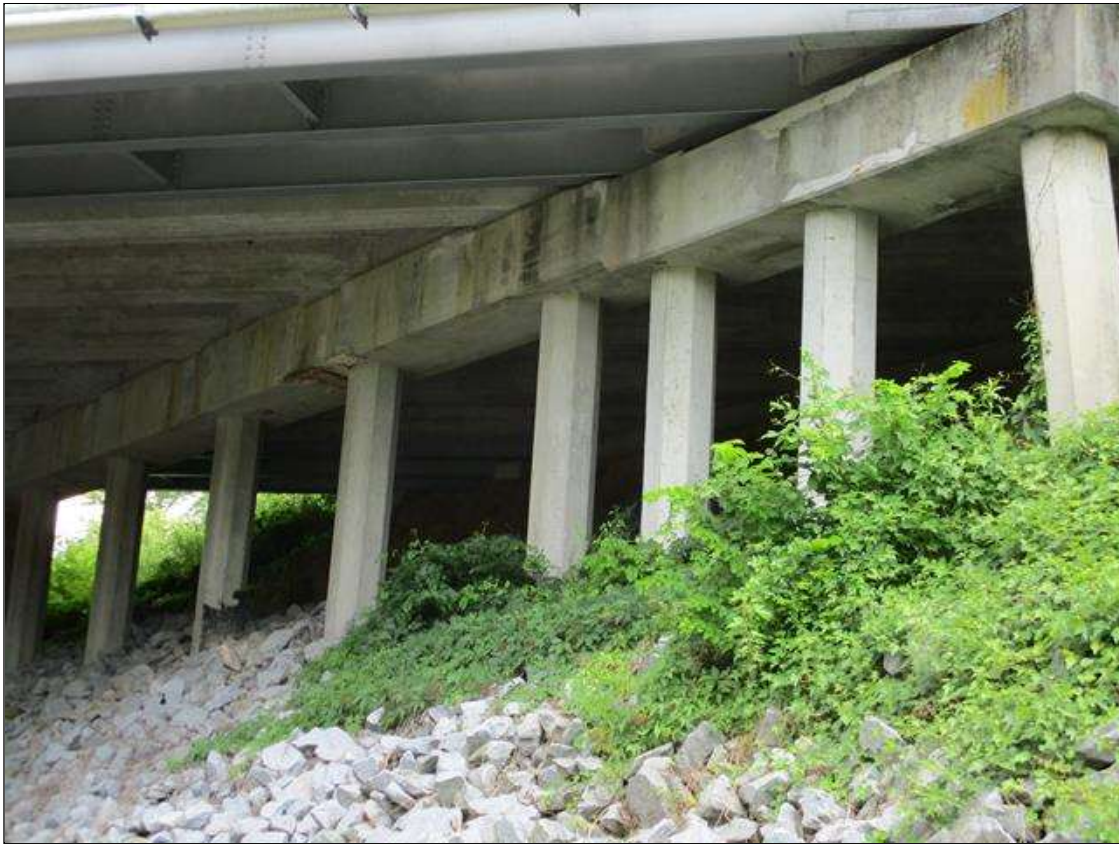
BENT 1 LOOKING SOUTH
