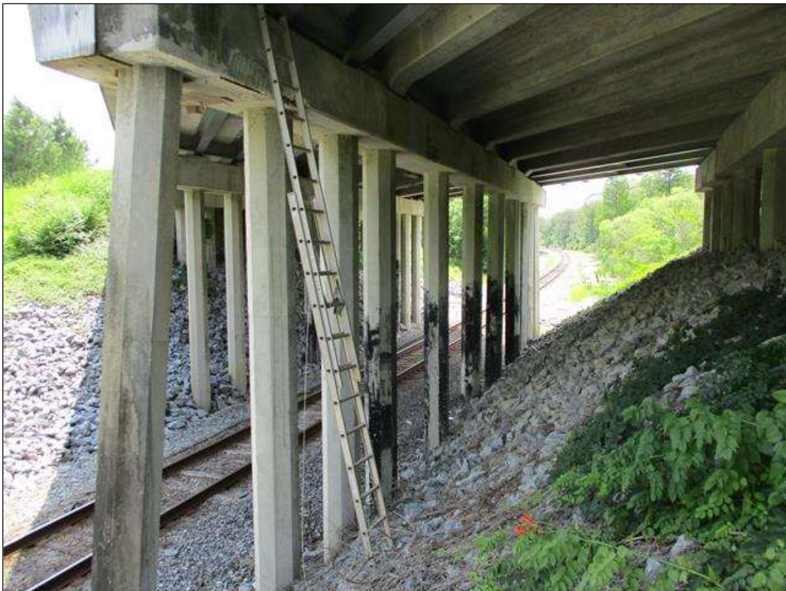
BENT 3 LOOKING SOUTH
