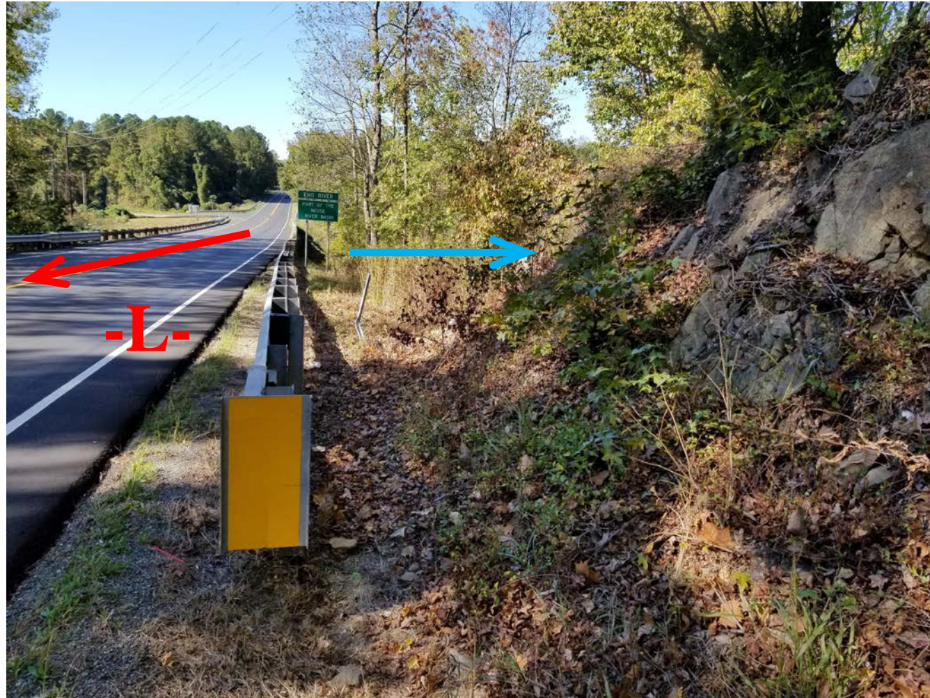
Standing near End Bent 2 facing toward End Bent 1
