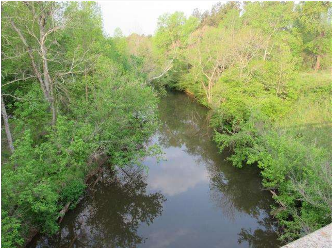
FROM BRIDGE LOOKING SOUTH UP STREAM
