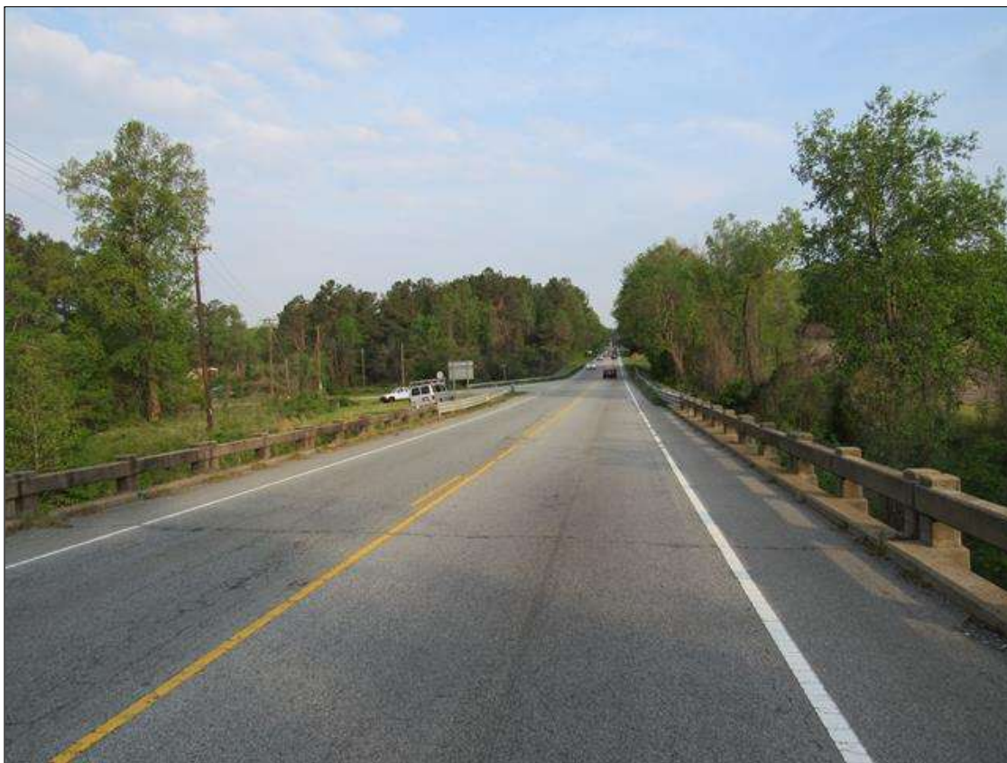
FROM BRIDGE LOOKING WEST
