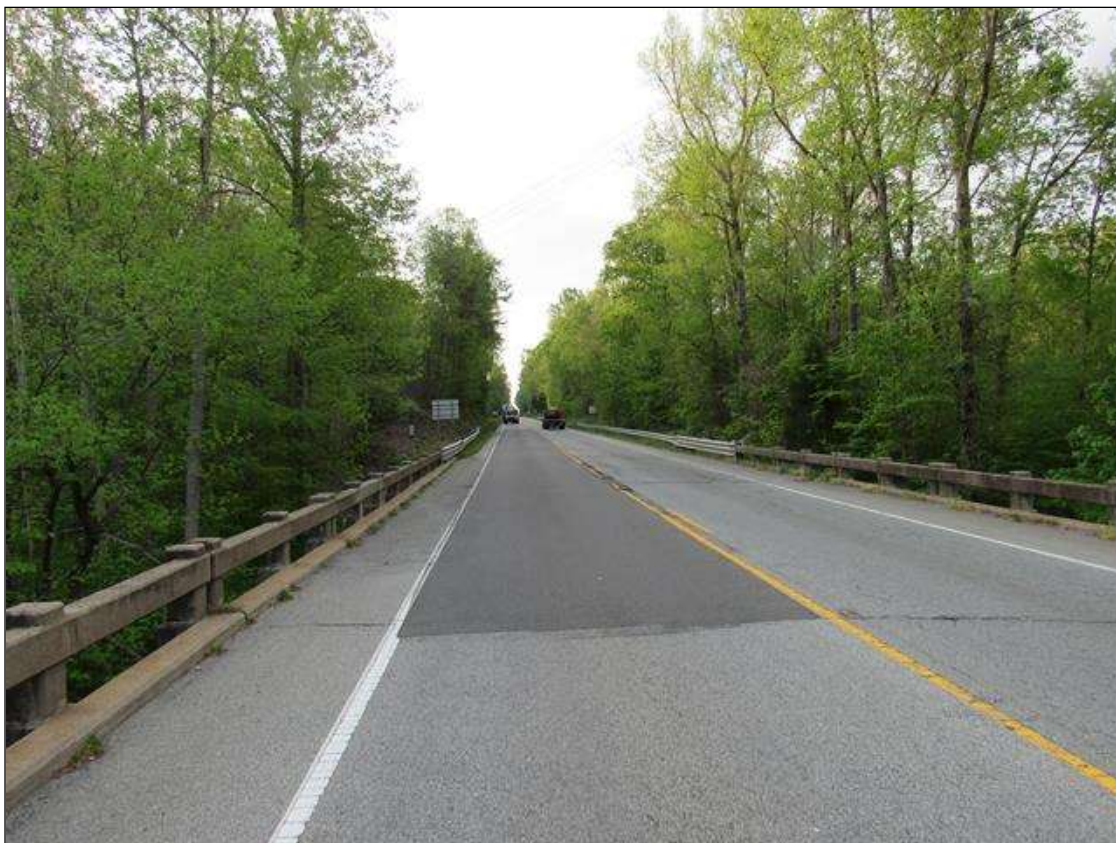
FROM BRIDGE LOOKING EAST
