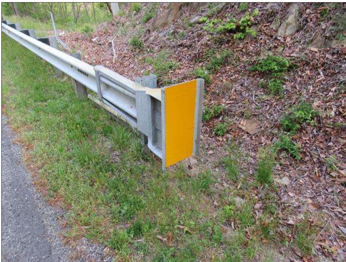
GUARD RAIL TERMINAL END
