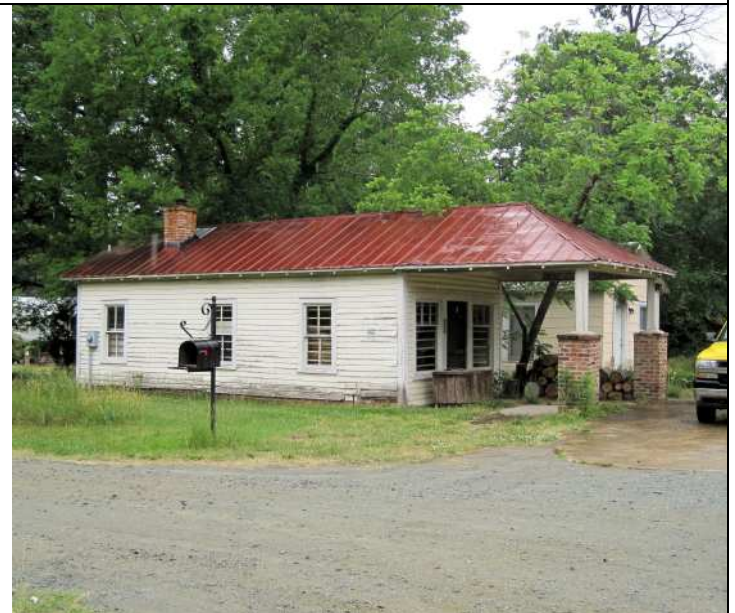
Site # 4: Former Gas Station. View to the northeast.
