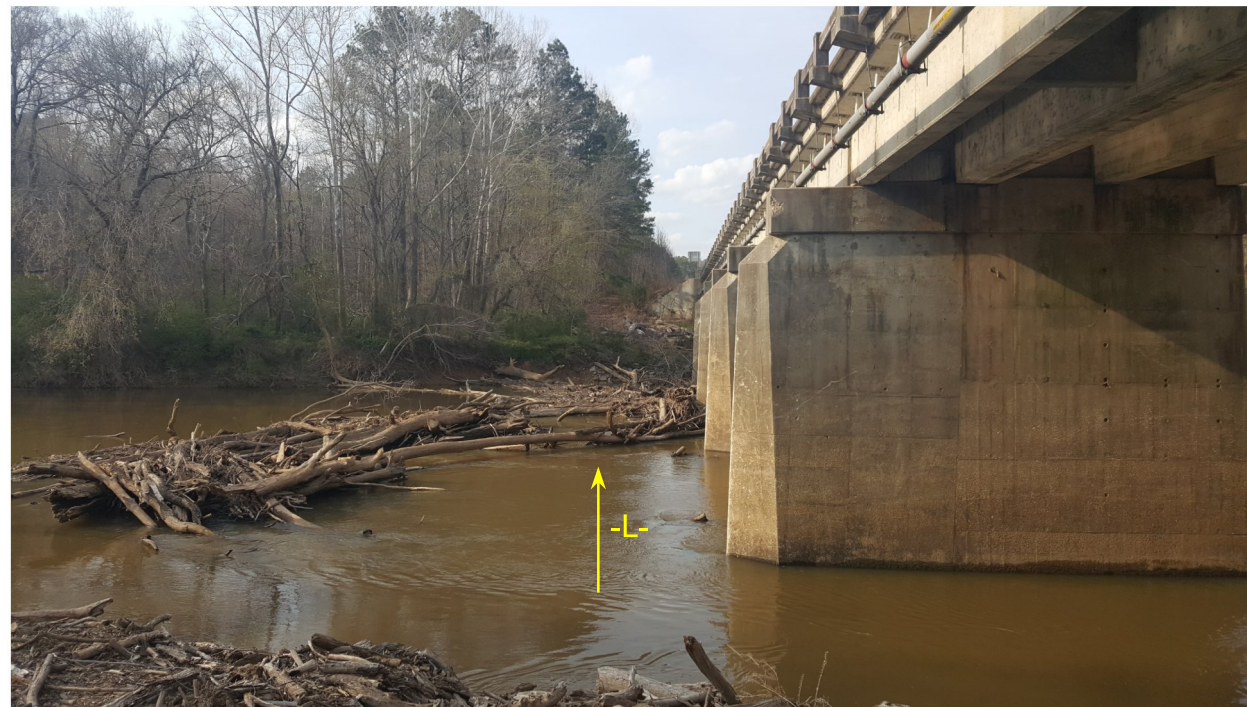
BENT 1 LOOKING UP STATION (NORTH)
