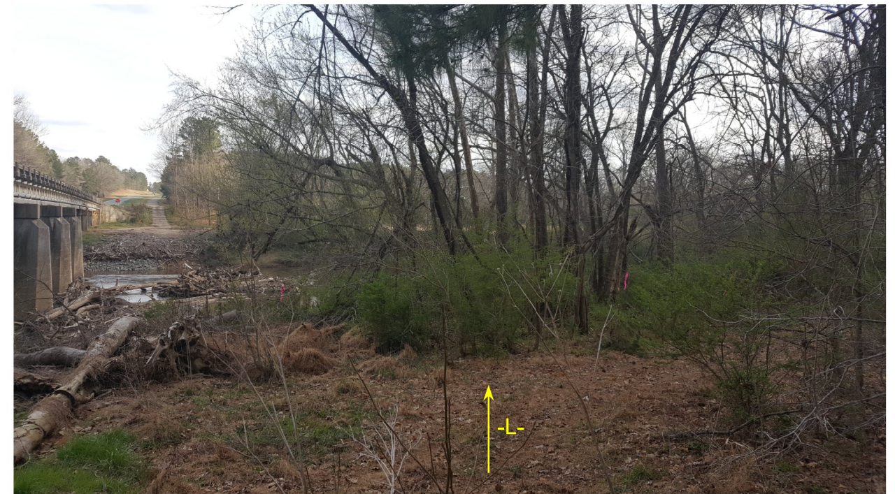
BENT 2 LOOKING DOWN STATION (SOUTH)
