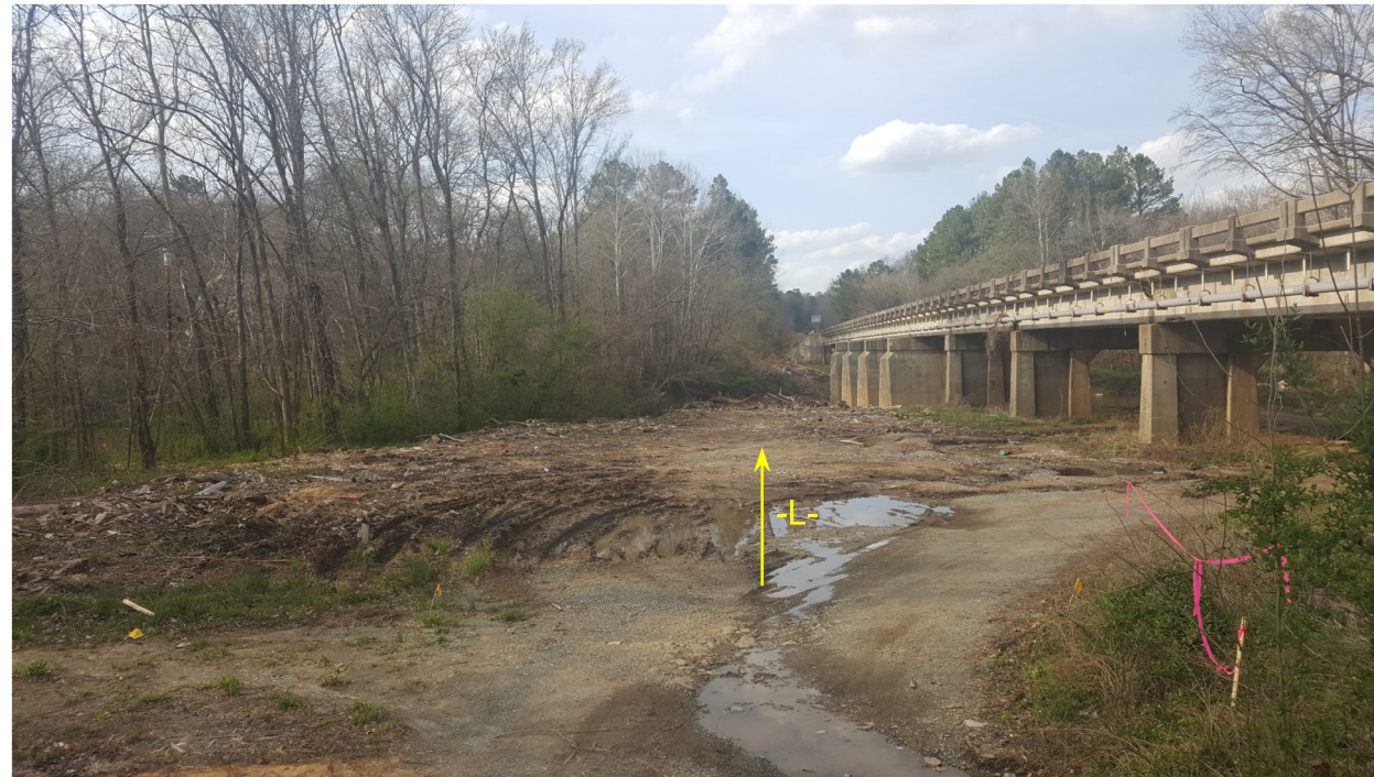
END BENT 1 LOOKING UP STATION (NORTH)
