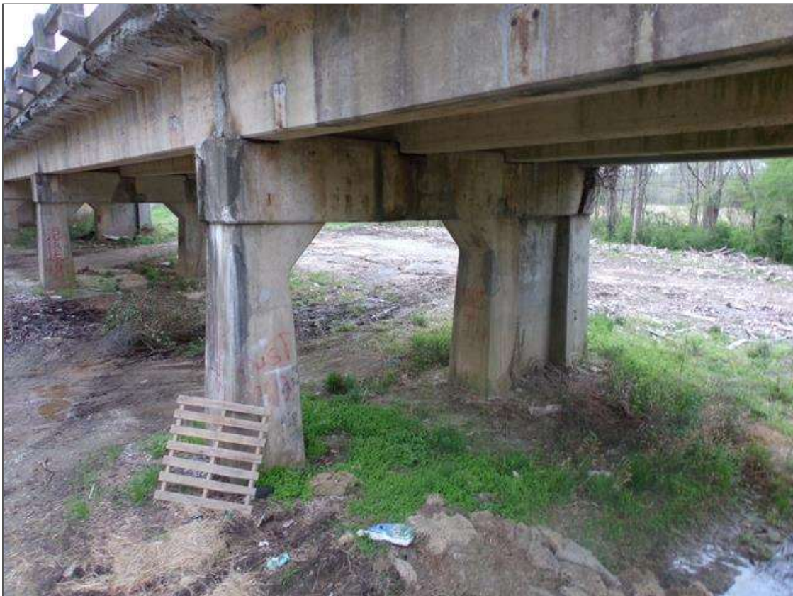
Pier 3, piers 1 and 2 similar
