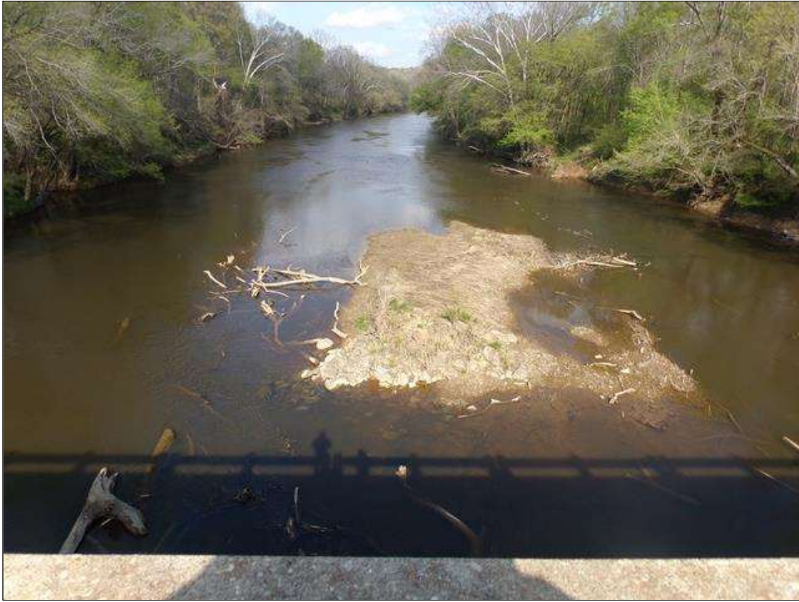
Looking east downstream
