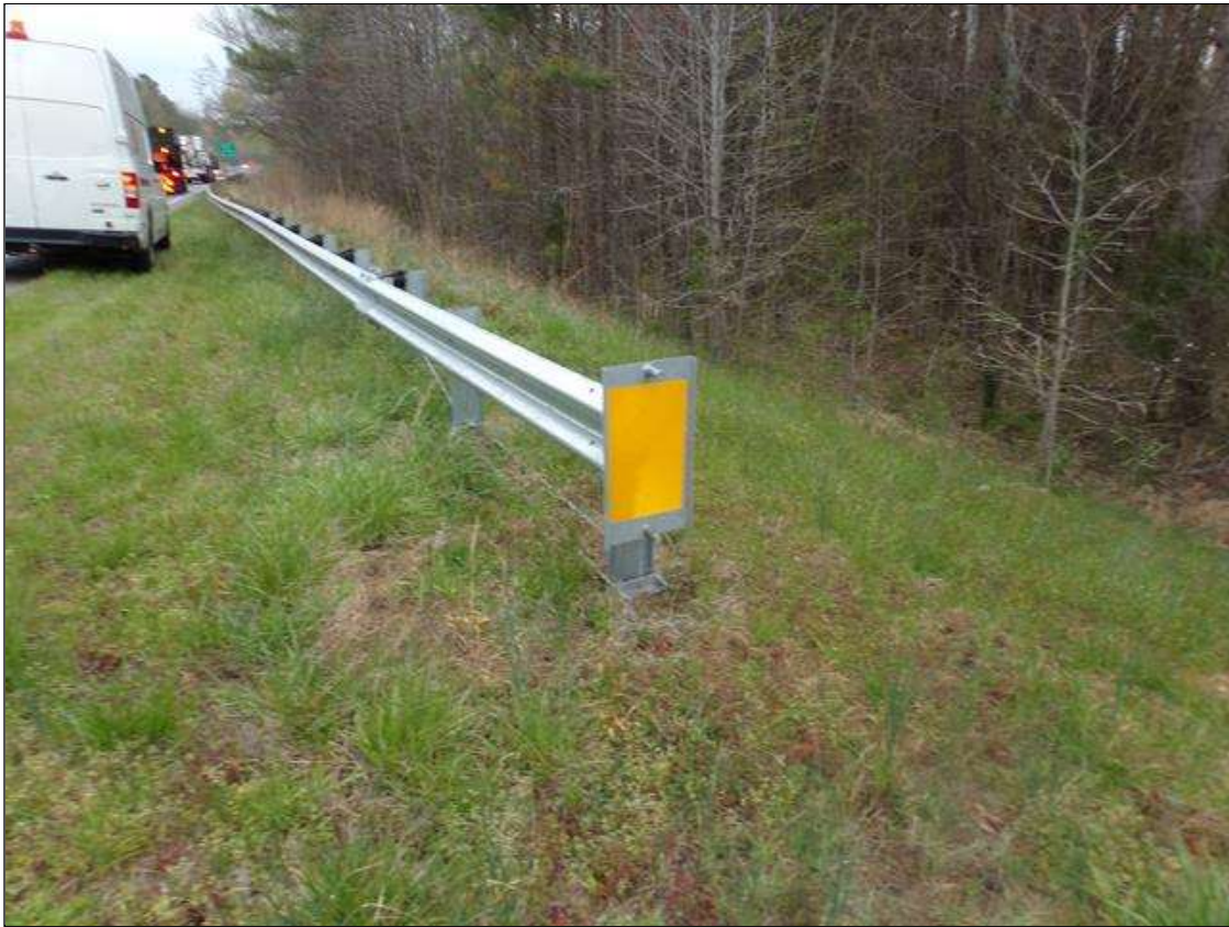
Guardrail terminal end southeast shown southwest similar
