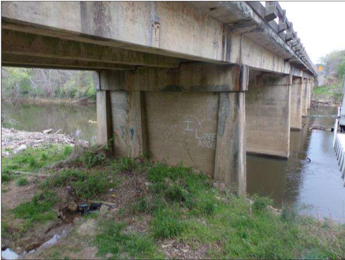
Pier 4, pier 9 similar
