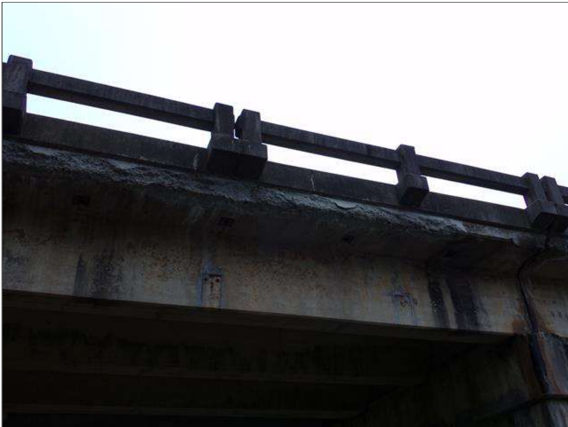
Span 4 Deck: Patched area 1' high x 6' long starting at pier 3 and 1' high x 25' long starting at pier 4 of east overhang that is distressed with efflorescence/stalactites/staining and cracking throughout.
