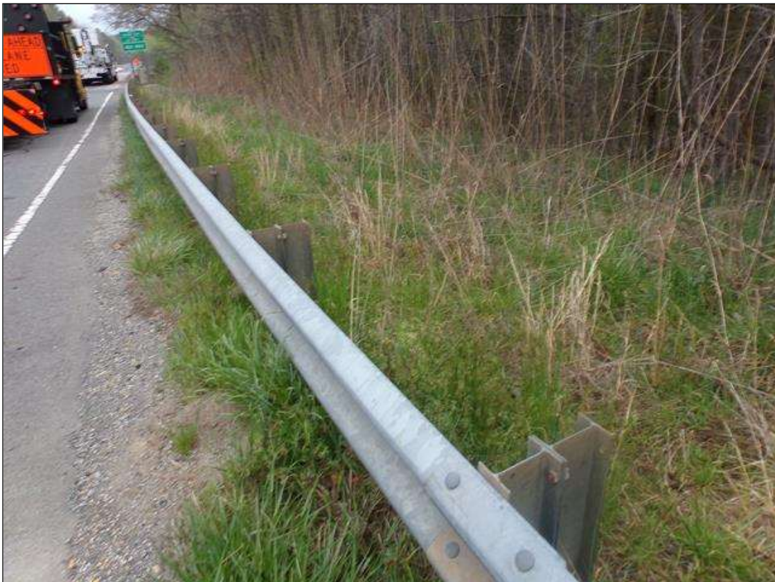
Guardrail post spacing midway southeast shown all others similar
