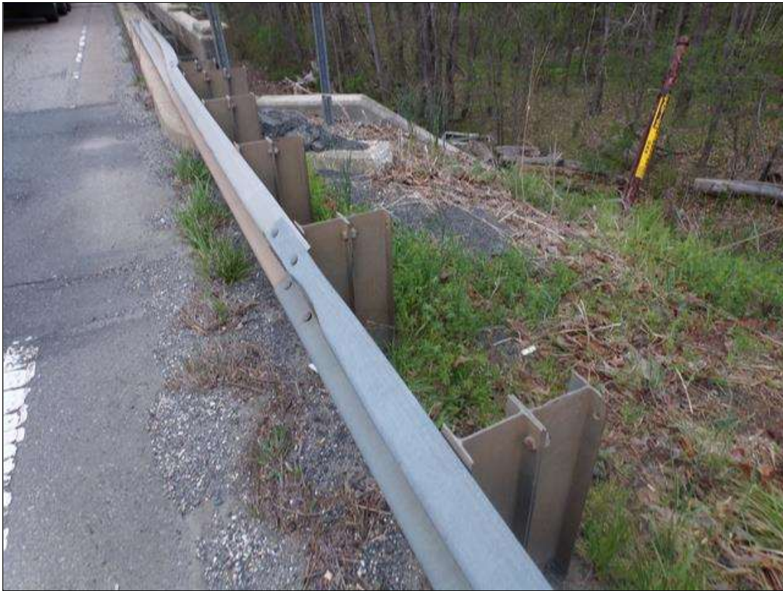
Guardrail post spacing at bridge southeast shown all others similar
