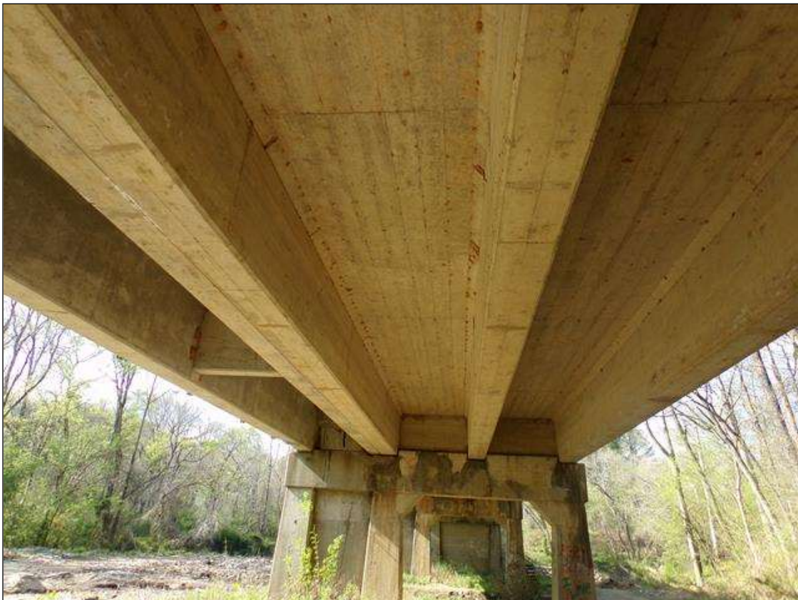
Superstructure underside span 2 shown, all others similar
