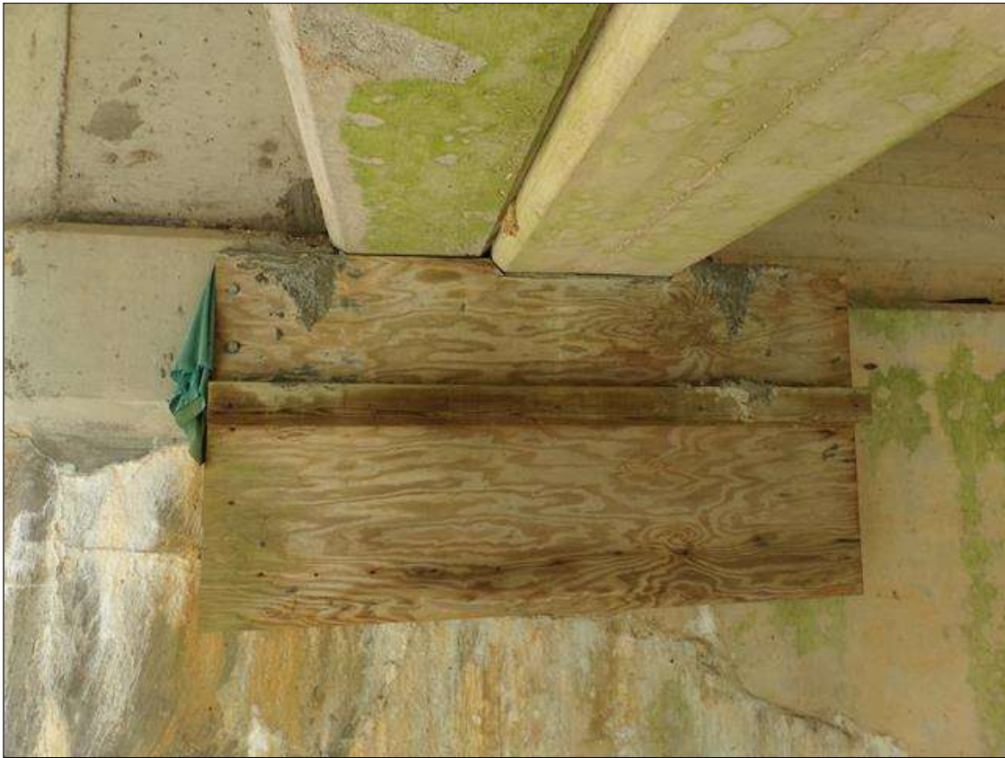
Form work left in place 4' long x 3' high under beams 2 and 3.
