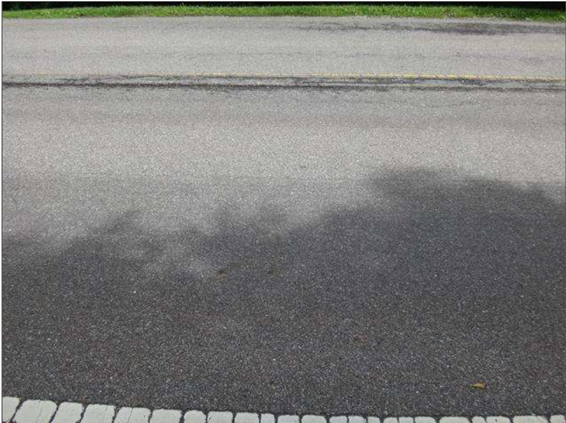
asphalt wearing surface over culvert
