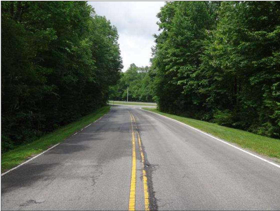
north approach looking south
