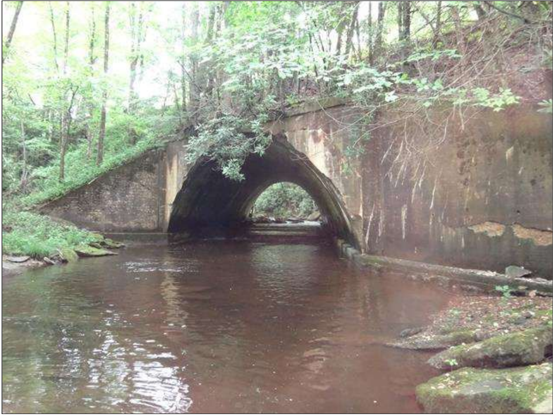
downstream profile looking east
