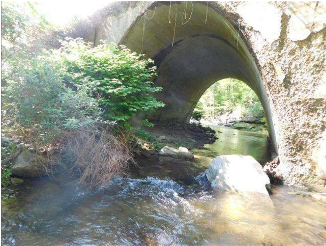
LOOKING WEST UPSTREAM THRU BARREL 1
