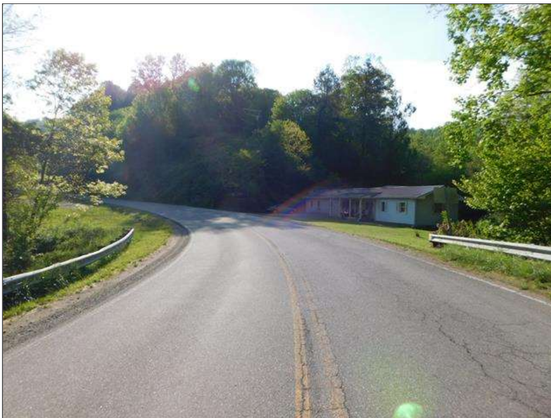
FROM STRUCTURE LOOKING SOUTH
