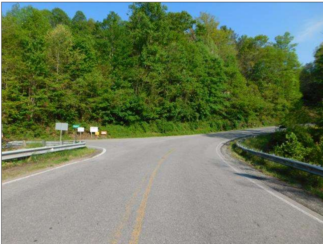
FROM STRUCTURE LOOKING NORTH
