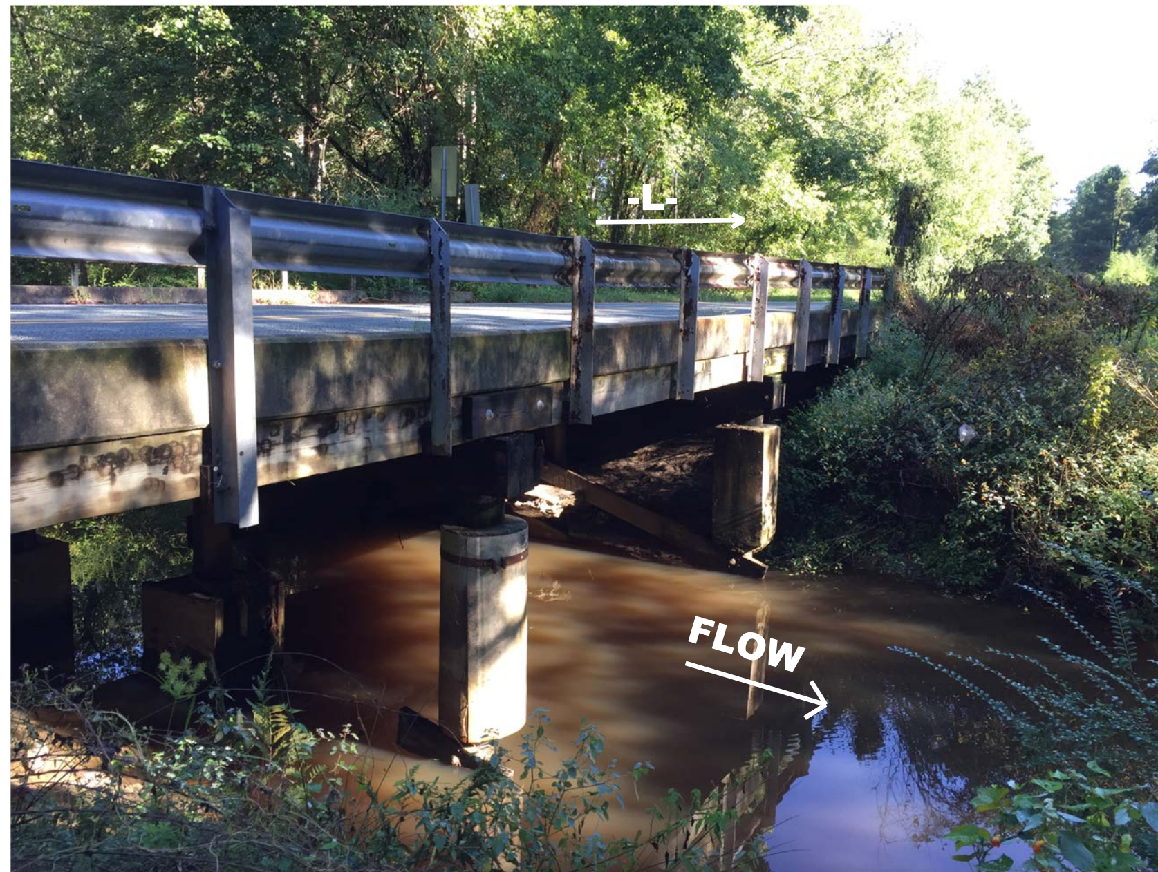
PHOTOGRAPH NO.1. VIEW LOOKING WEST.
