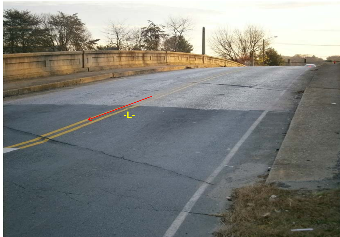
View Looking West along -L- from End Bent 2
