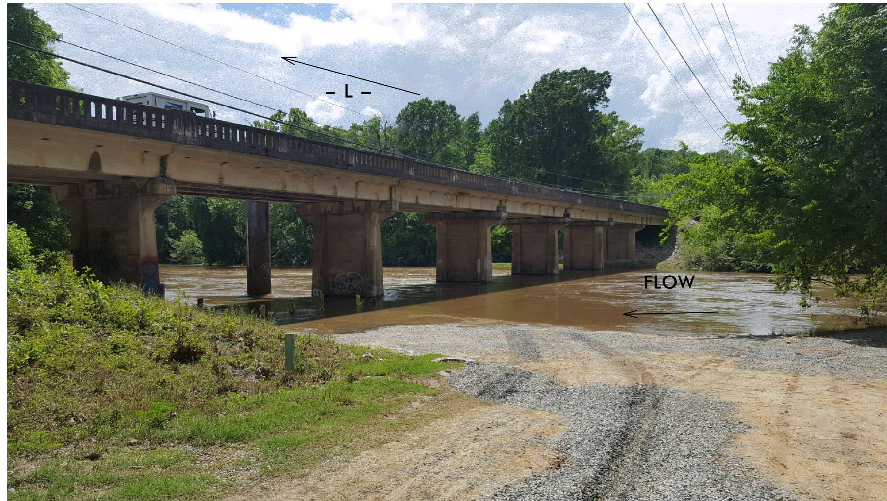
Looking west toward End Bent 1
