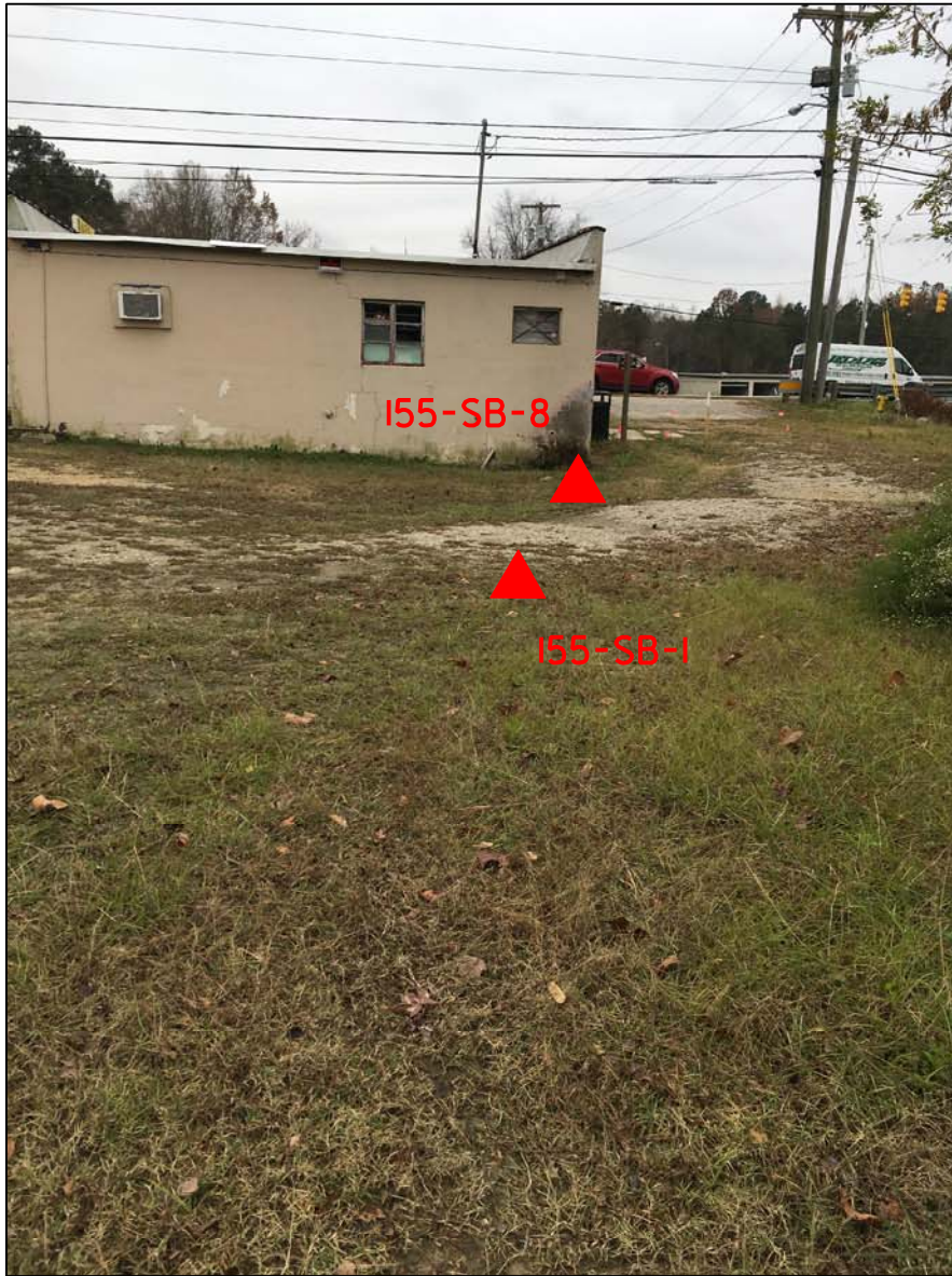
PHOTO 3 - VIEW OF SOIL BORINGS LOOKING SOUTH
