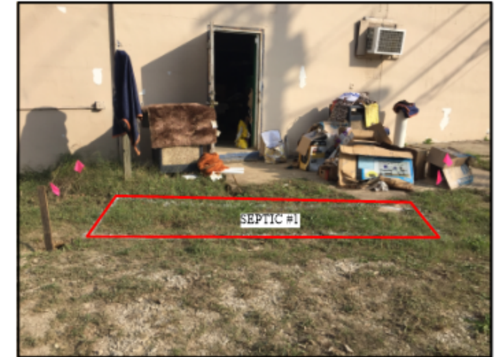
LOCATION OF NORTH SEPTIC TANK #1
