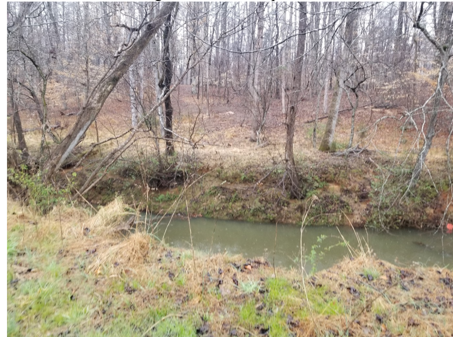
Photo 4: Looking Northeast towards End Bent 2 (Mill Creek flows from right to left)
