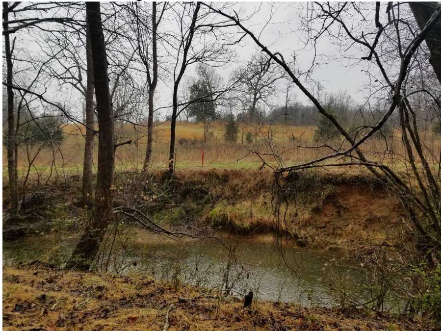
Photo 3: Looking Southwest towards End Bent 1 (Mill Creek flows from left to right)
