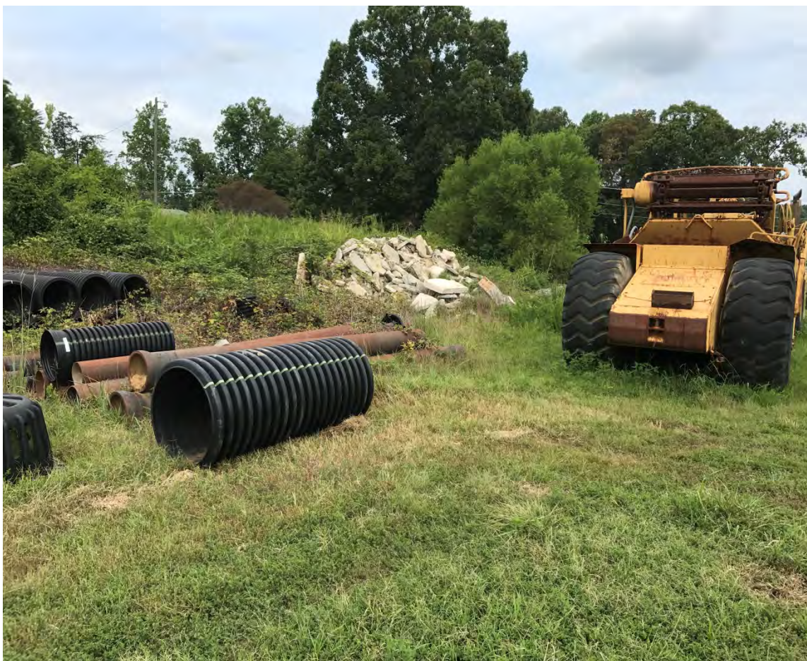
Photograph No. 3 View of grading equipment and construction materials on site.
