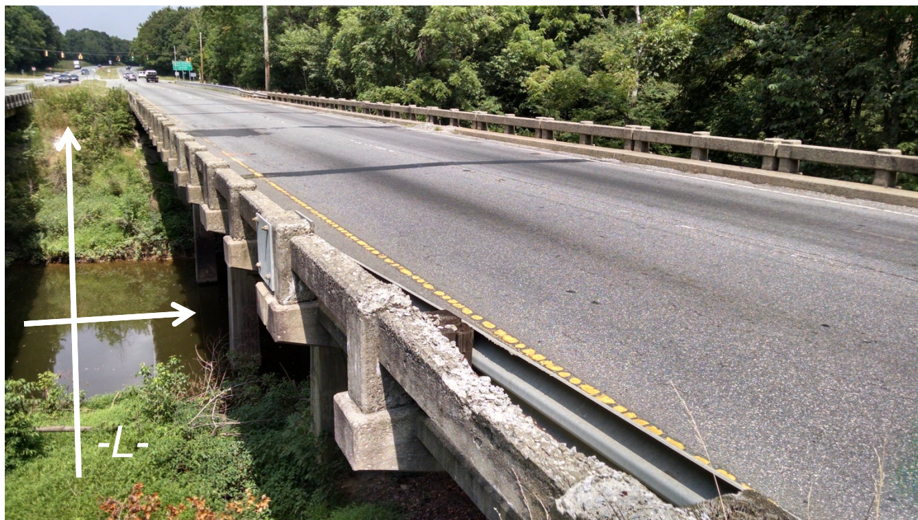
BRIDGE NO. 237 FACING NORTH EAST
