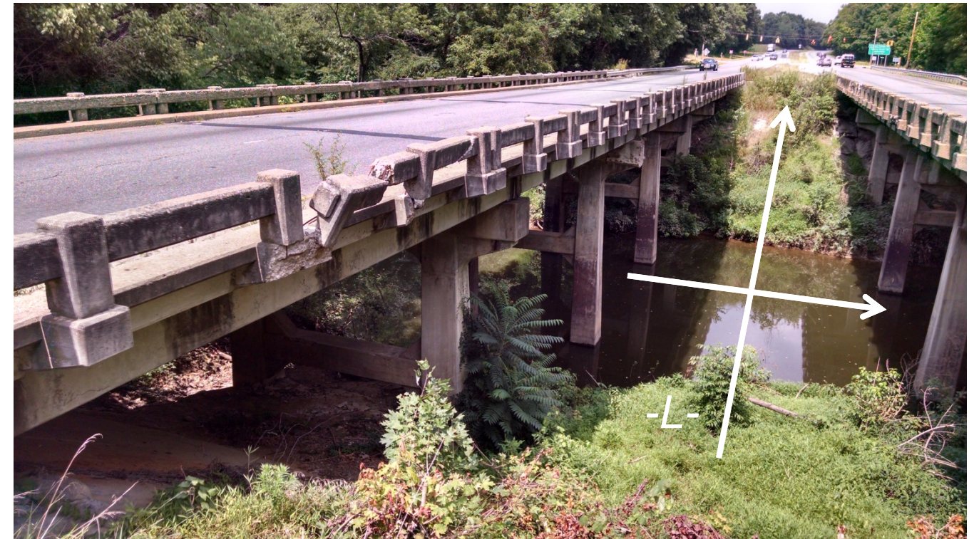
BRIDGES NO. 237 & 242 FACING NORTH EAST
