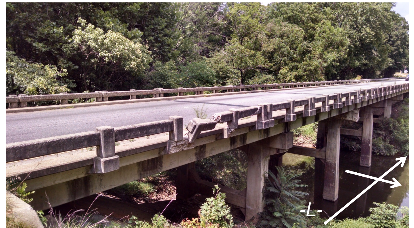
BRIDGE NO. 242 FACING NORTH EAST
