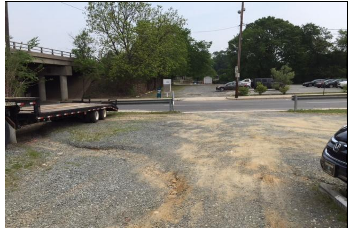
PHOTOGRAPH NO. 4: WEST APPROACH TO END BENT NO.2 ON -S2- ALIGNMENT, LOOKING EAST
