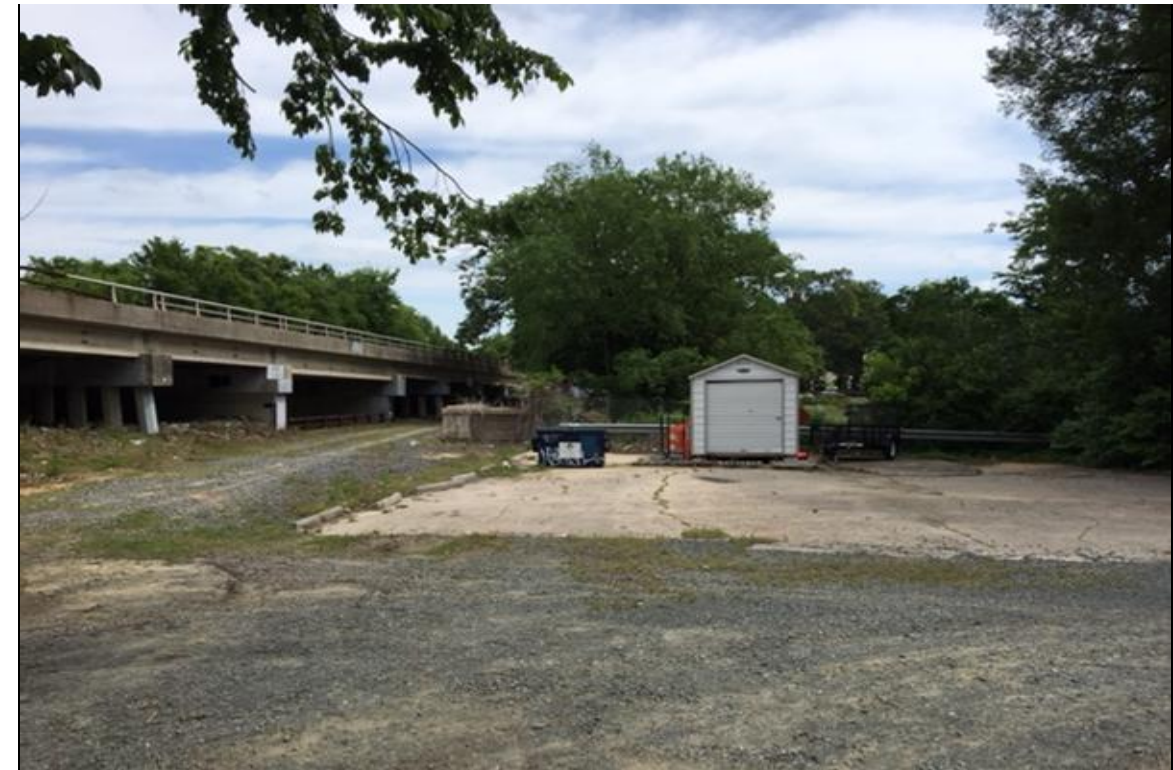
PHOTOGRAPH NO. 4: WEST APPROACH TO END BENT NO.2 ON -S1- ALIGNMENT, LOOKING EAST
