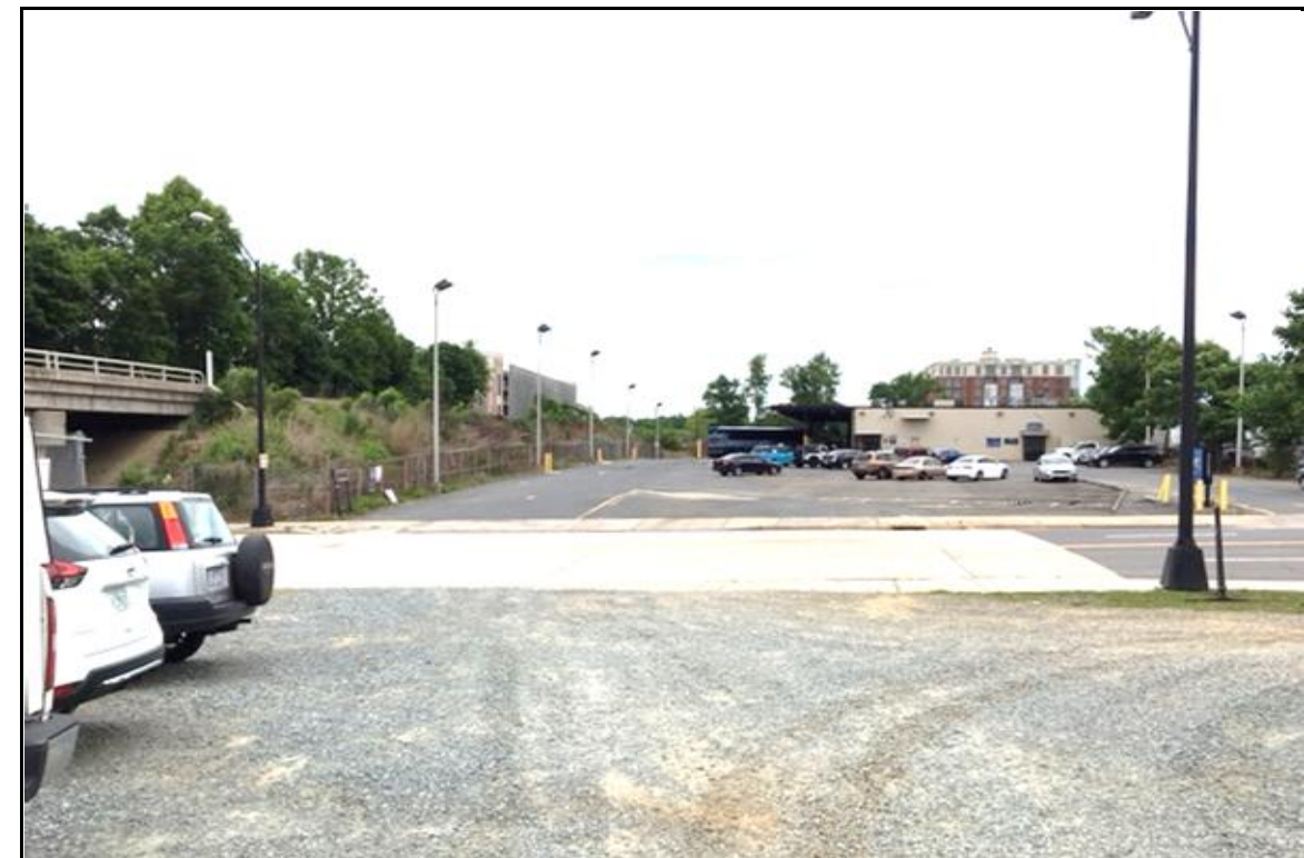
PHOTOGRAPH NO. 4: WEST APPROACH TO END BENT NO.2 ON -S1- ALIGNMENT, LOOKING EAST
