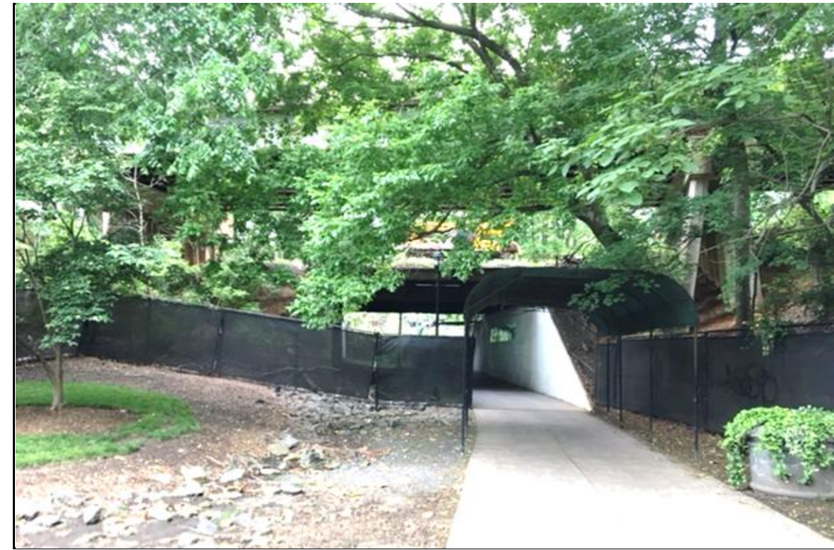
PHOTOGRAPH NO. 3: ON TUNNEL WALKWAY, NORTHWEST OF -A1- ALIGNMENT, LOOKING SOUTHEAST
