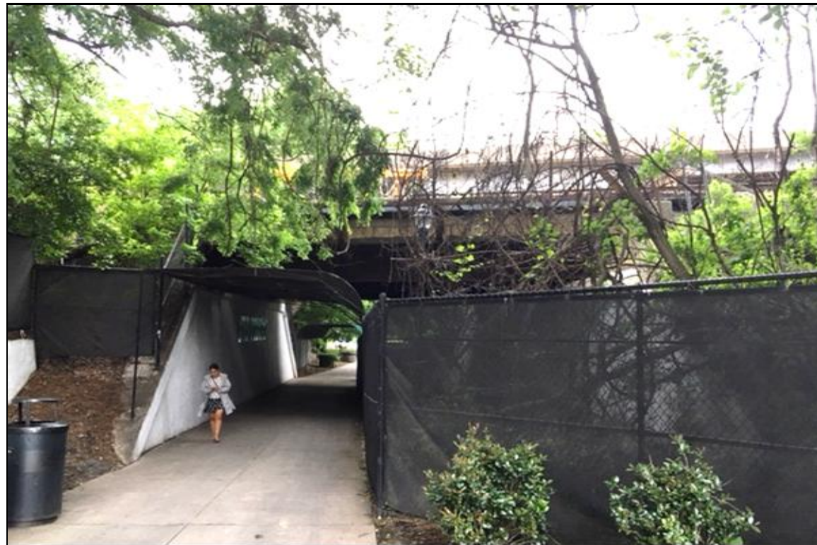
PHOTOGRAPH NO. 2: ON TUNNEL WALKWAY, SOUTHEAST OF -A1- ALIGNMENT, LOOKING NORTHWEST
