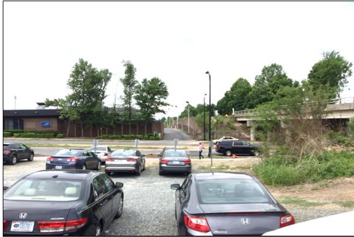
PHOTOGRAPH NO. 1: EAST APPROACH TO END BENT NO. 1 ON -S1- ALIGNMENT, LOOKING WEST
