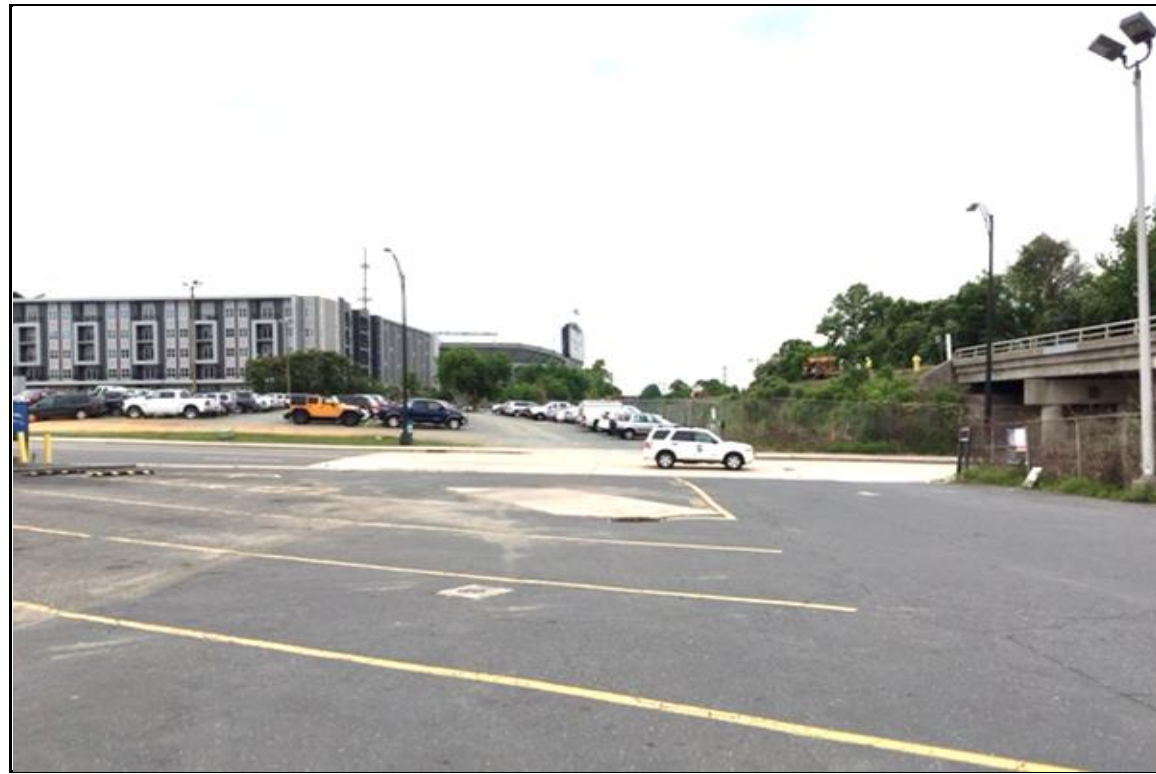
PHOTOGRAPH NO. 1: EAST APPROACH TO END BENT NO. 1 ON -S1- ALIGNMENT, LOOKING WEST
