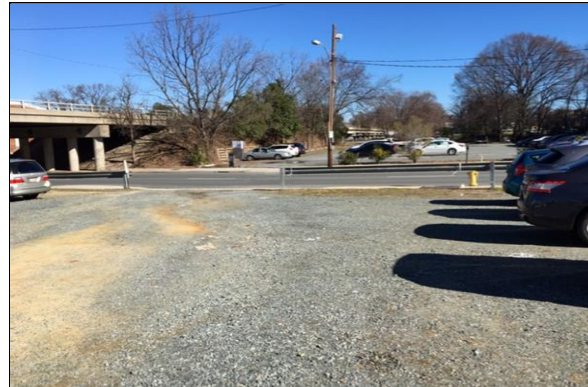
PHOTOGRAPH NO. 4: WEST APPROACH TO END BENT NO.2 ON -S1- ALIGNMENT, LOOKING EAST
