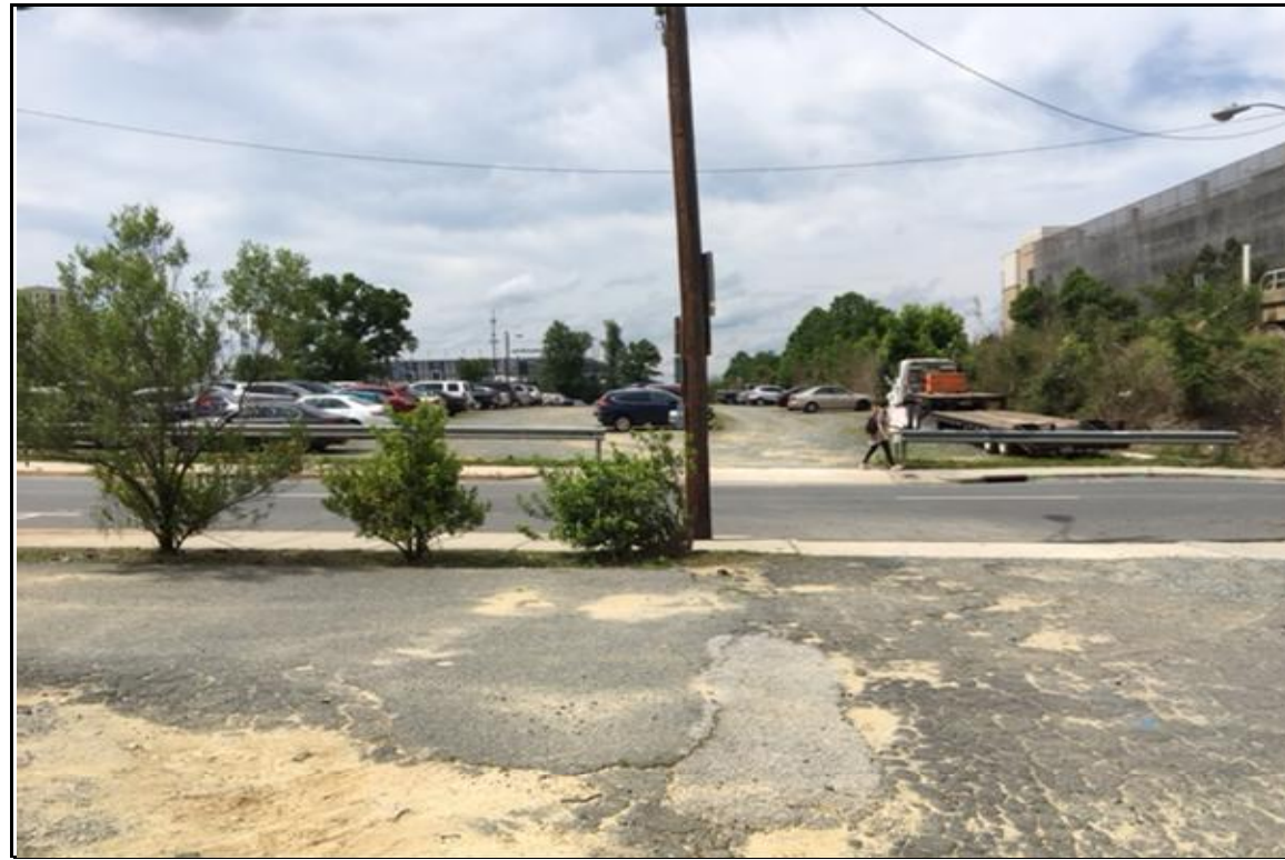
PHOTOGRAPH NO. 1: EAST APPROACH TO END BENT NO. 1 ON -S1- ALIGNMENT, LOOKING WEST
