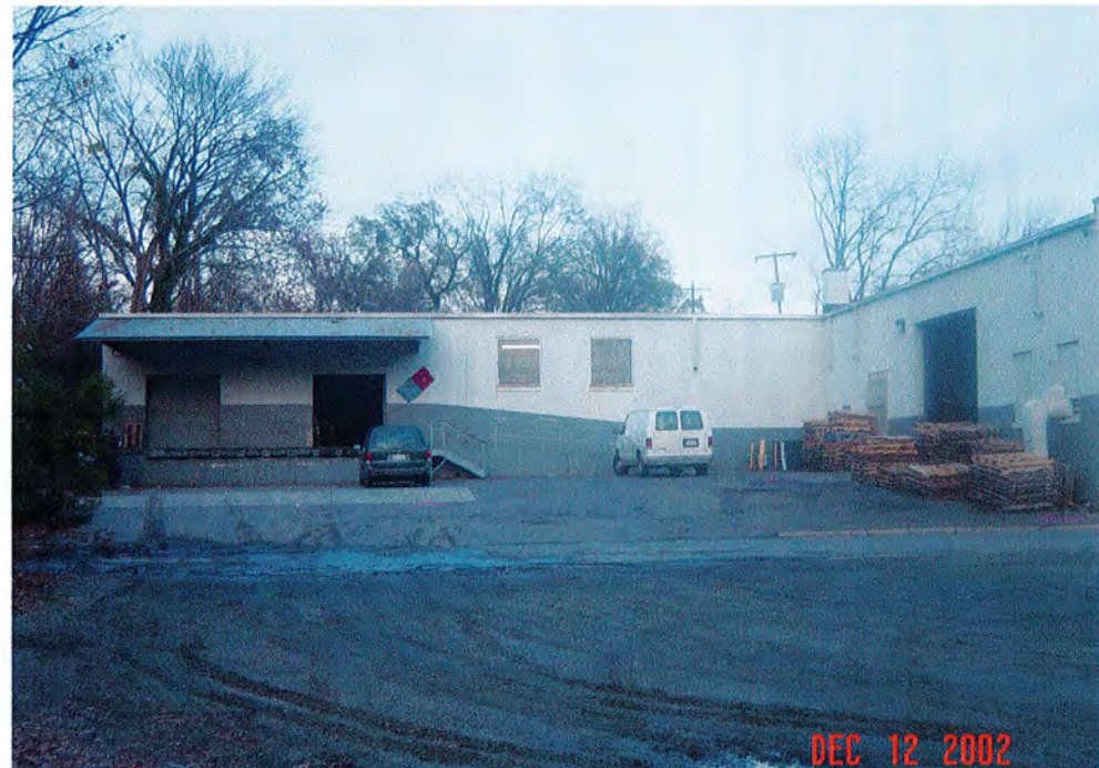
(NORTHEASTWARD VIEW) PHOTO SHOWS THE LOADING DOCK AREA LOCATED ALONG HEARN PLACE.
