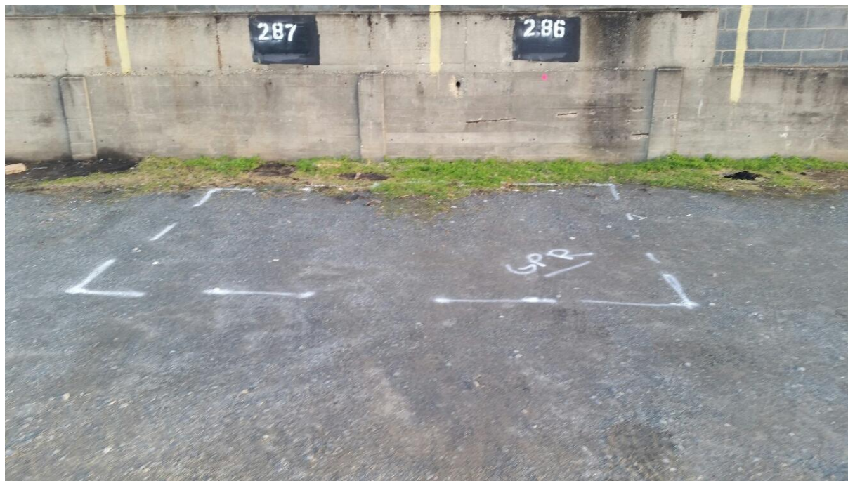
Photo 11: Showing GPR anomaly in Parcel 10.
