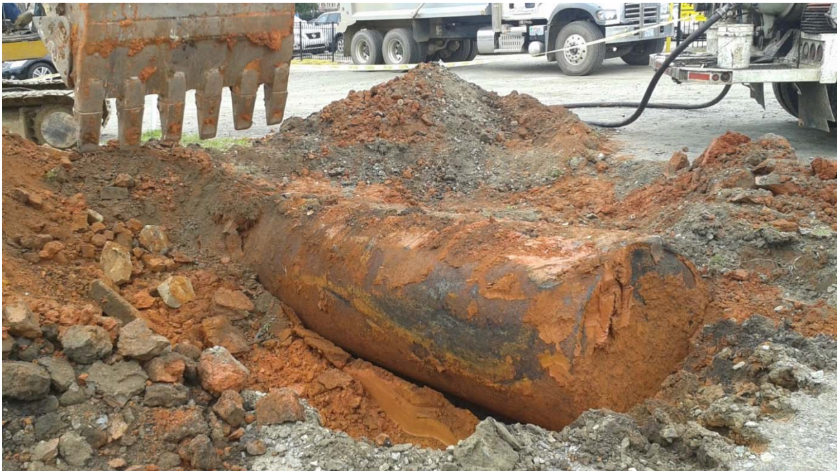
Photograph 2: View of heating oil tank removed from the southern portion of the property.
