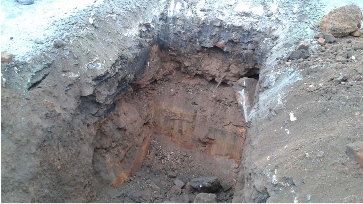
Photograph 1: View of excavation area in the central portion of the property.
