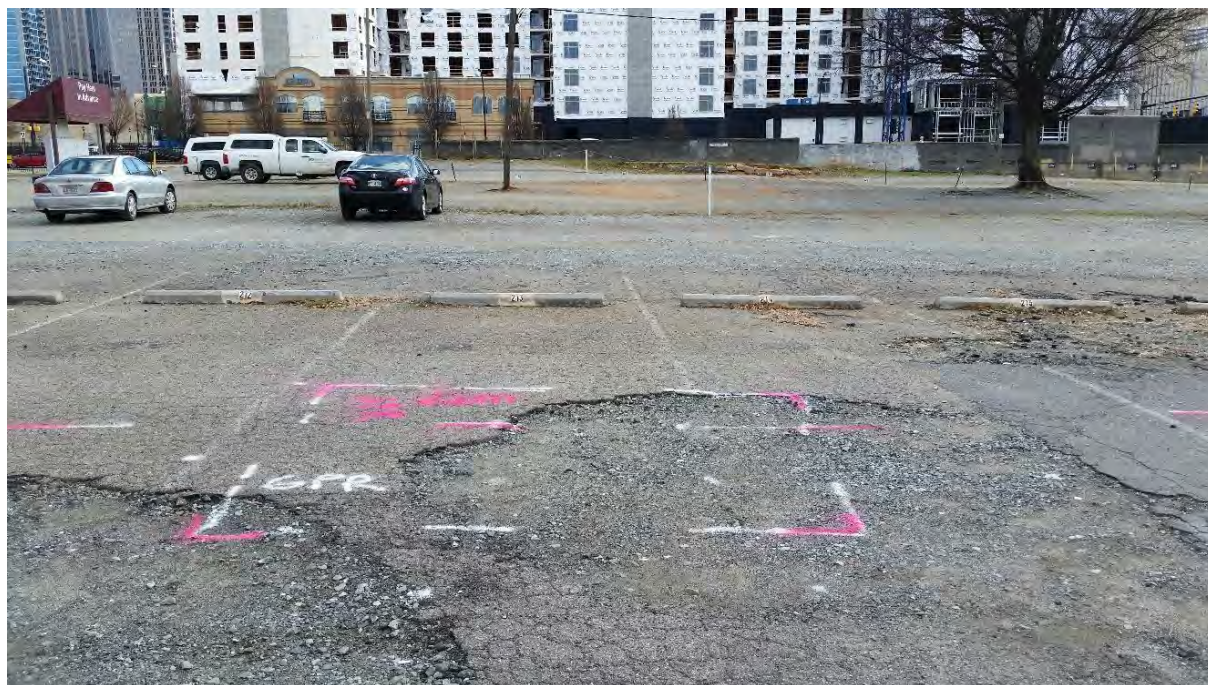
Photo 12: Showing "Possible UST" in Parcel 4B.
