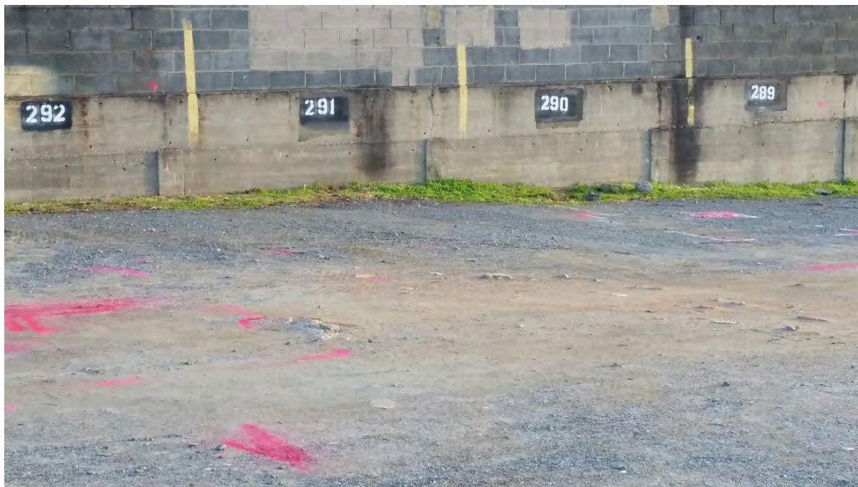
Photo 7: Looking south towards Parcel 10.
