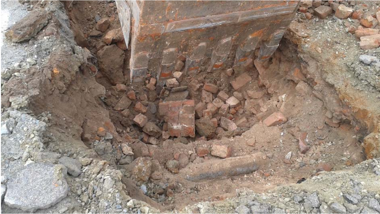
Photograph 1: View of brick and metal piping debris in excavation.
