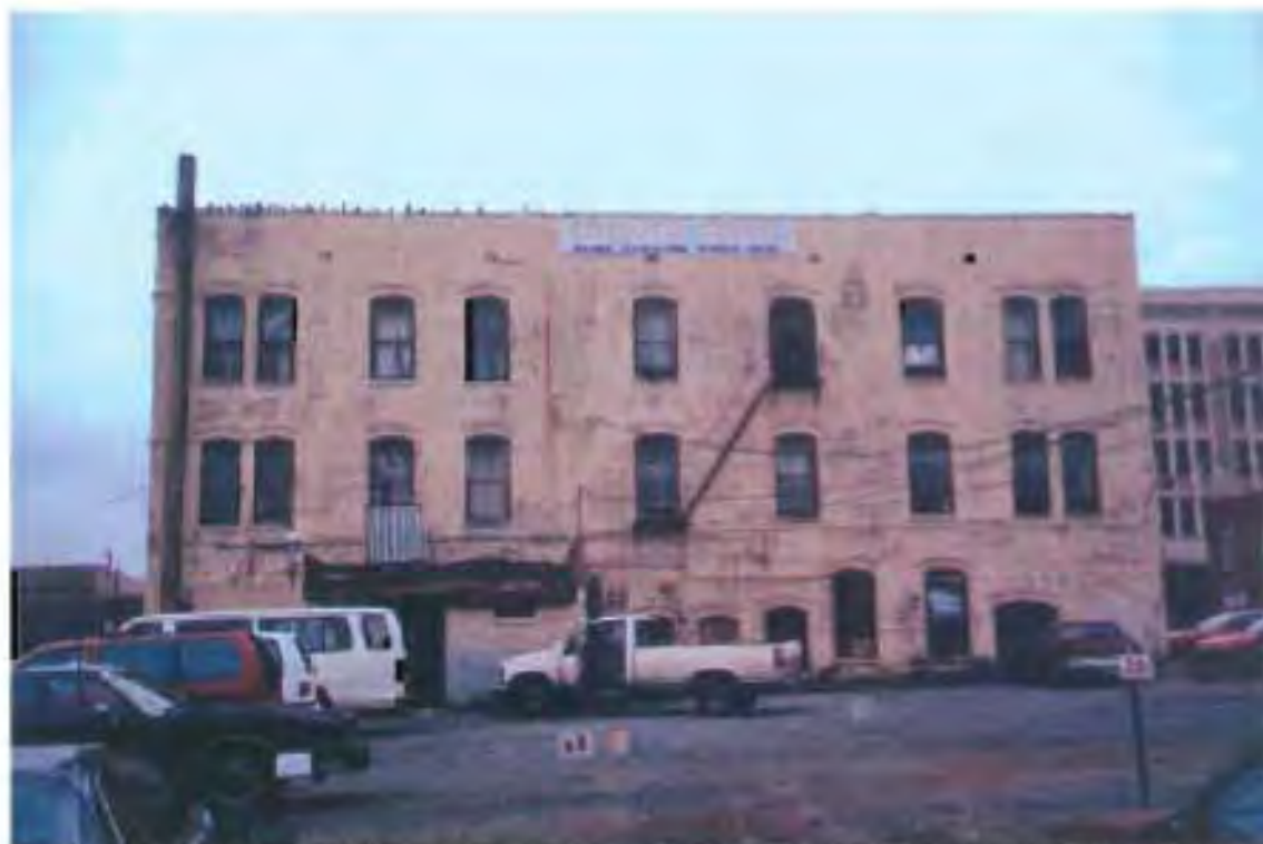
Property #26 and #27. 525 West Trades Street, Travelers Hotel, Presto Grill and 533 West Trade Street, Paid Parking, respectively.
