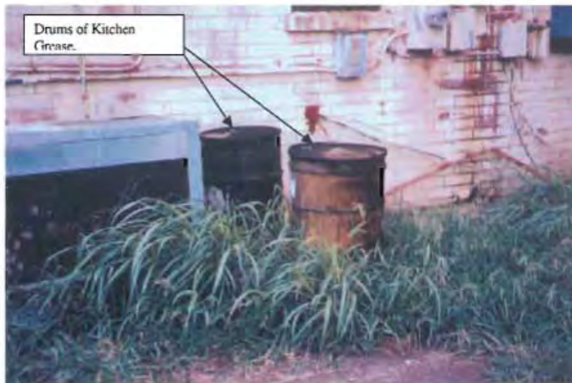
Property #26. 525 West Trades Street, Travelers Hotel and Presto Grill, back side of building.
