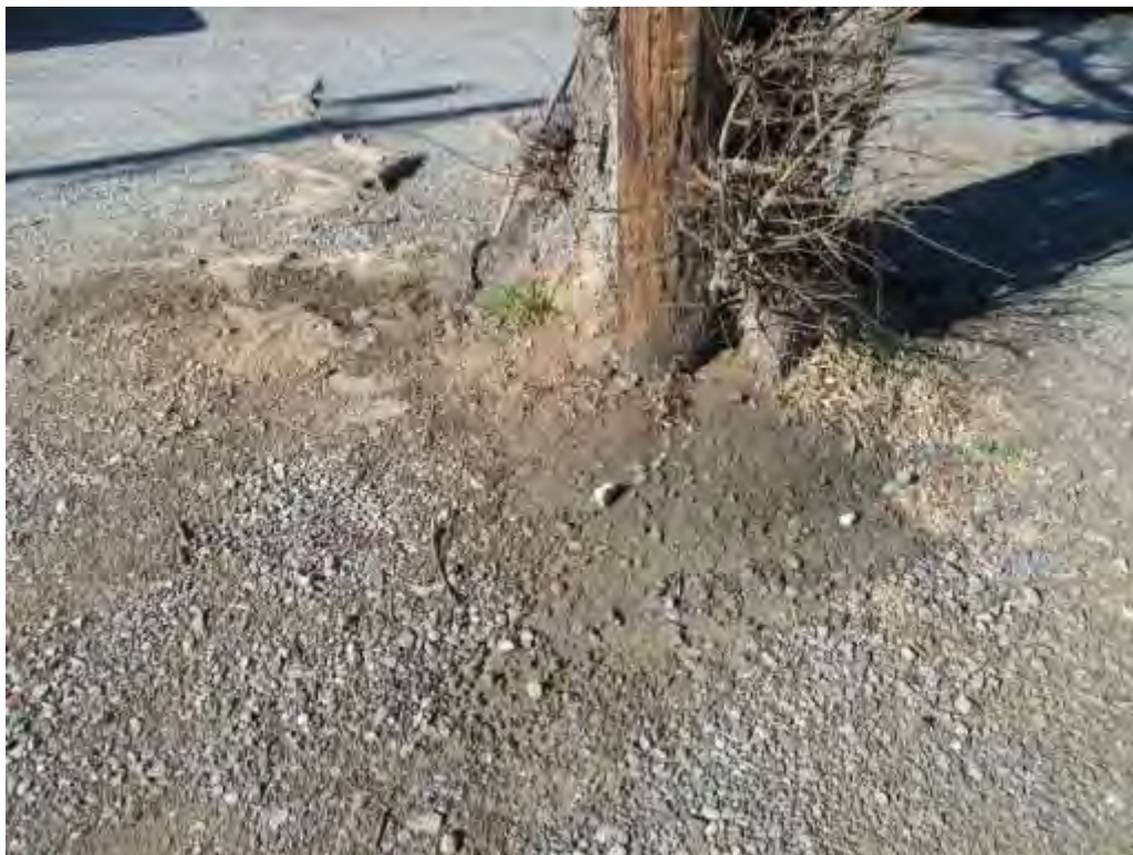
Photo 8 View of de minimis oil stains at the base of tree and light pole.
