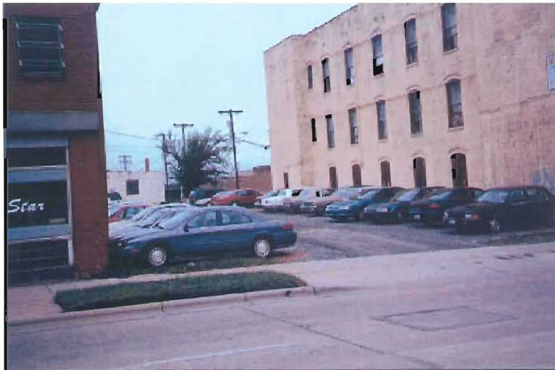
Property #32. 517 West Trade Street, Gravel Parking.
