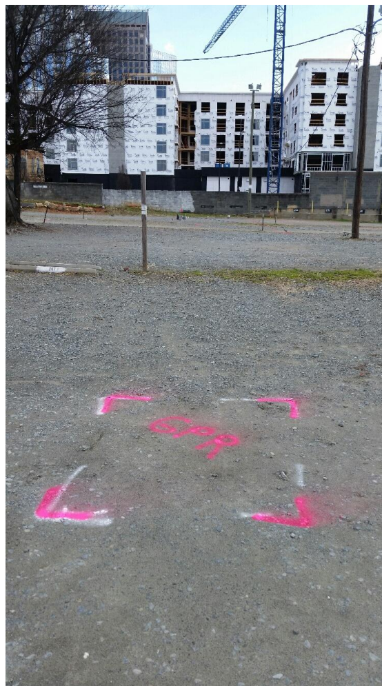
Photo 17: Showing GPR anomaly in Parcel 5B.
