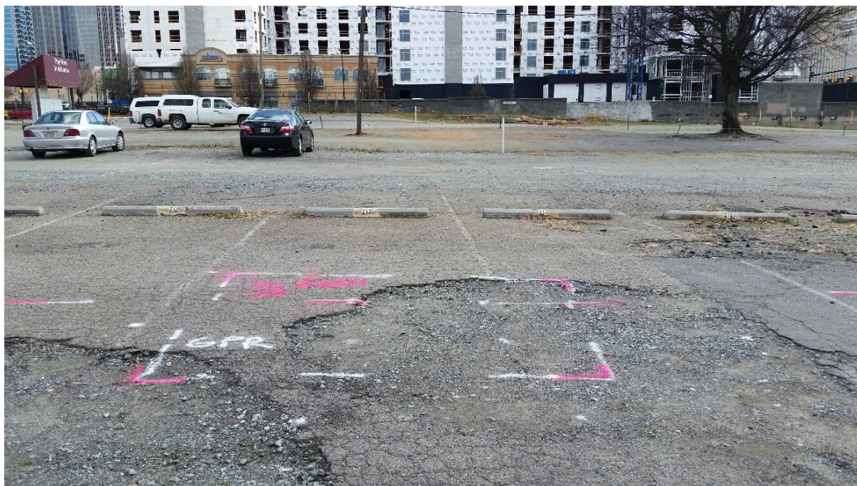
Photo 12: Showing "Possible UST" in Parcel 4B.
