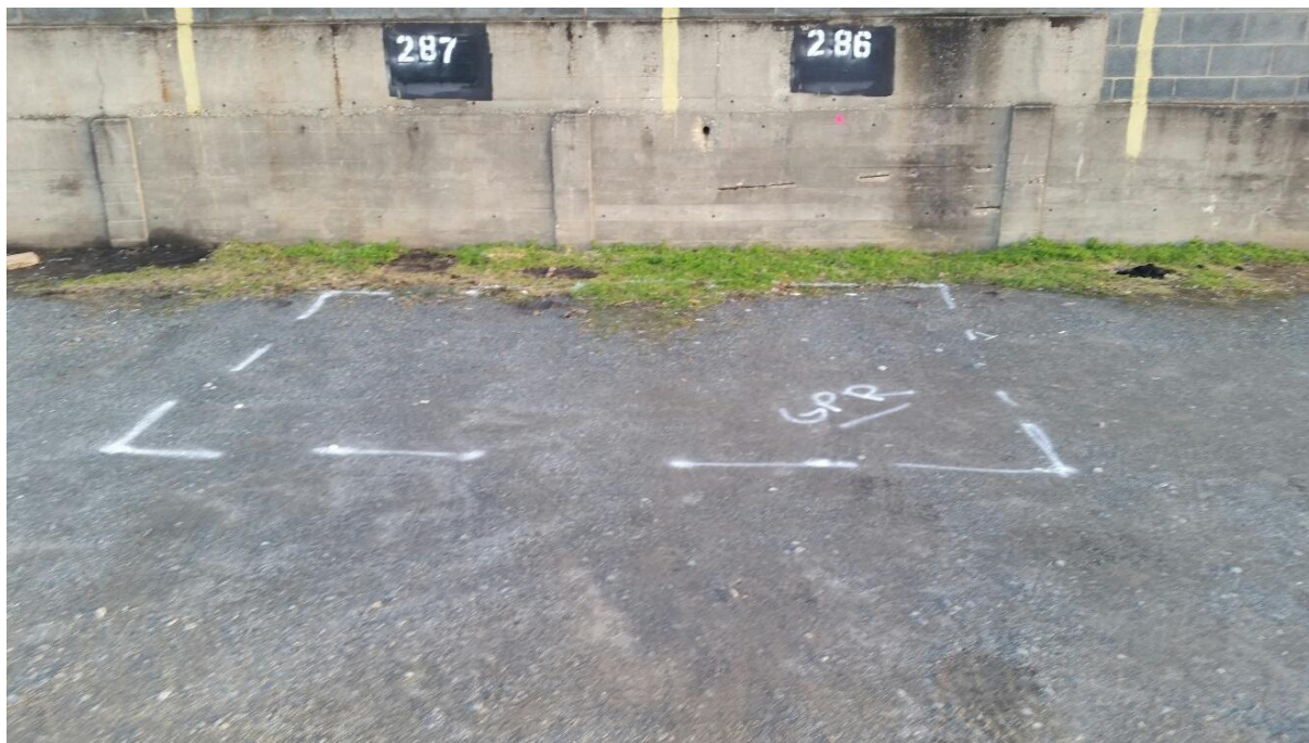
Photo 11: Showing GPR anomaly in Parcel 10.
