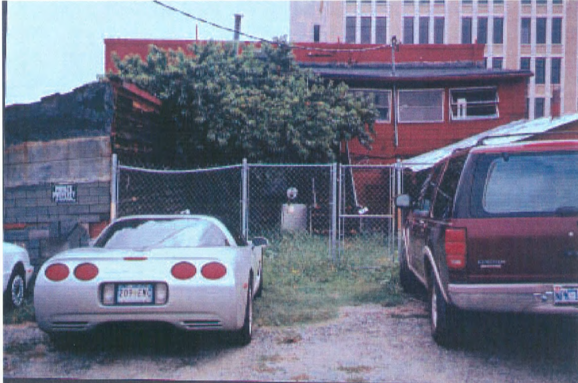
Property #33. 511 West Trade Street. Former Dirty Laundry Cleaners (from behind).
