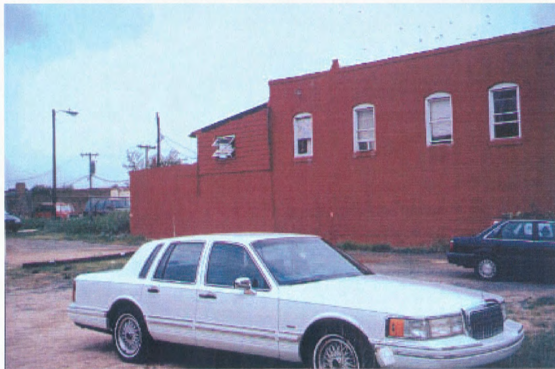
Property #33. 511 West Trade Street. Former Dirty Laundry Cleaners.
