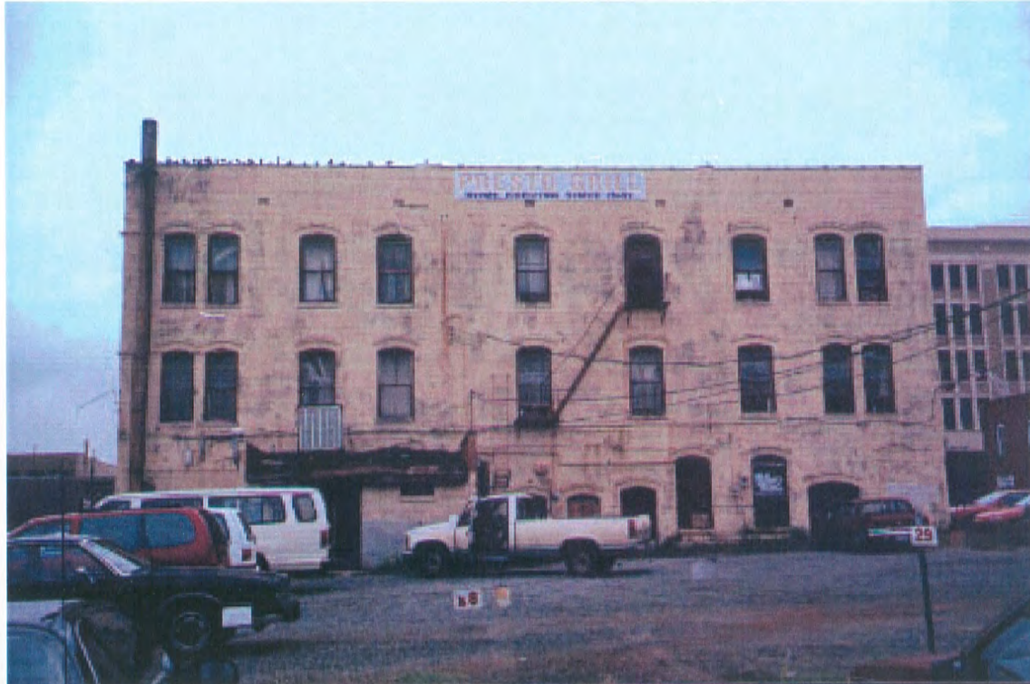
Property #26 and #27. 525 West Trades Street, Travelers Hotel, Presto Grill and 533 West Trade Street, Paid Parking, respectively.
