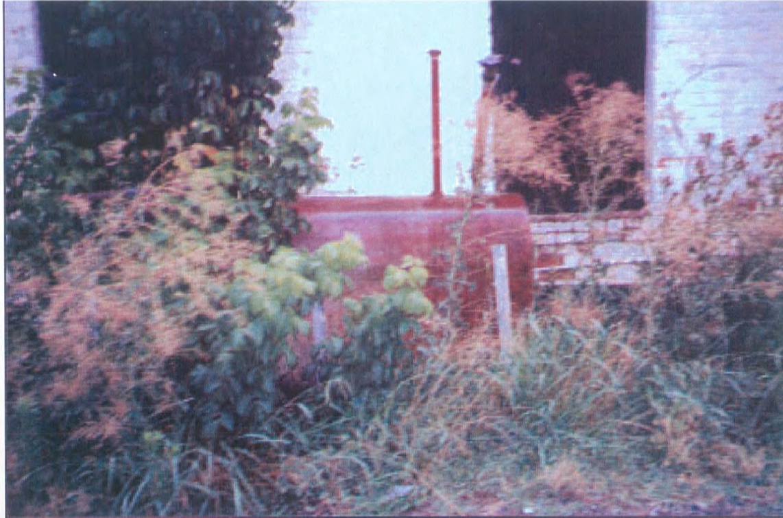
Property #30. 510 West 4 th Street, Former Heritage Printers (AST behind building).
