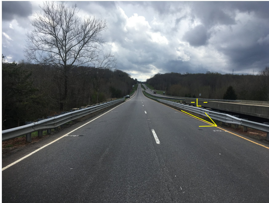
Photo No. 1: View at End Bent 2 looking south (downstation) on -L- (US 220 Bypass)
