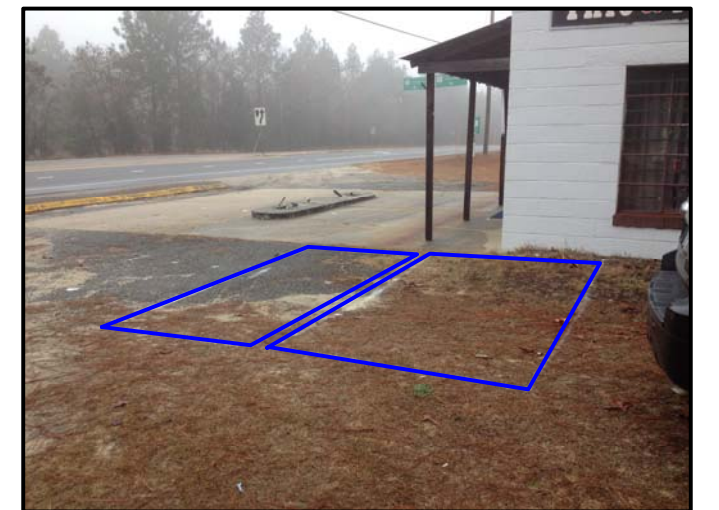
Area containing two possible USTs
