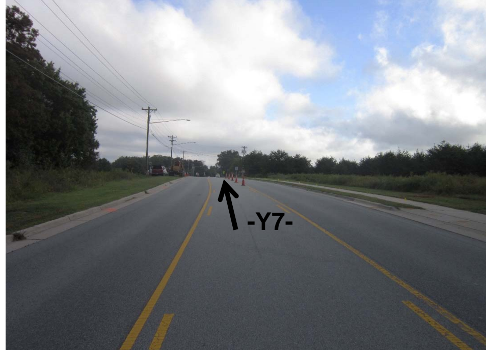
View looking upstation along proposed bridge alignment
