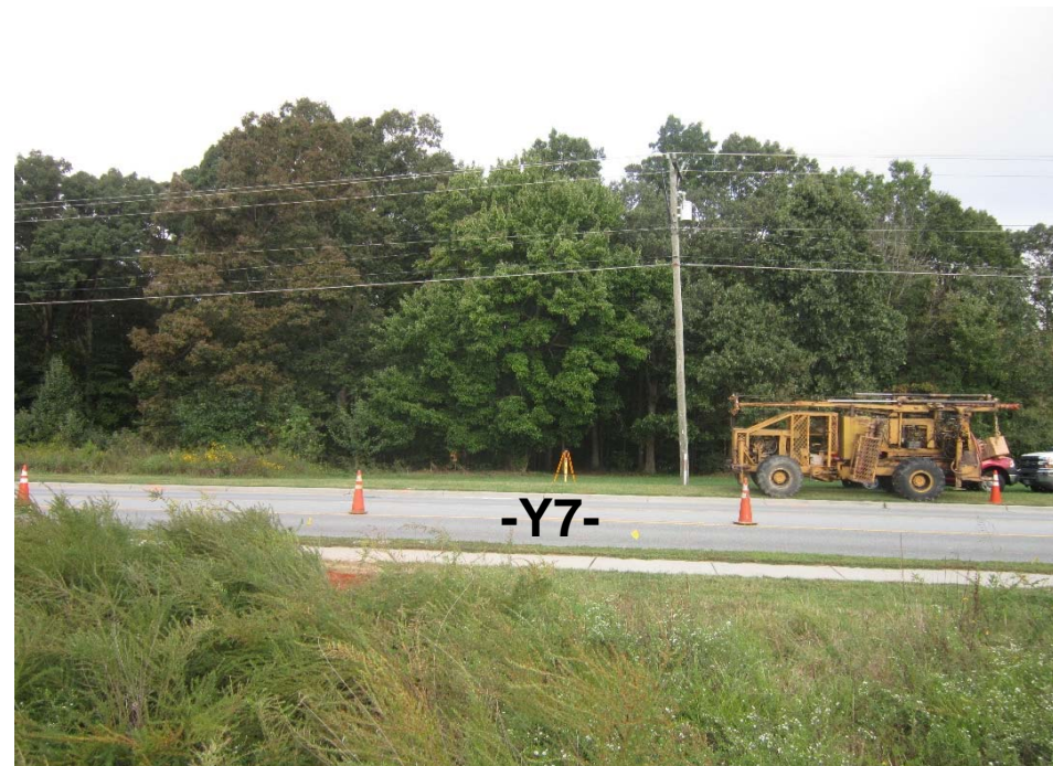
View looking nearly perpendicular to proposed bridge alignment (approximate northwest)
