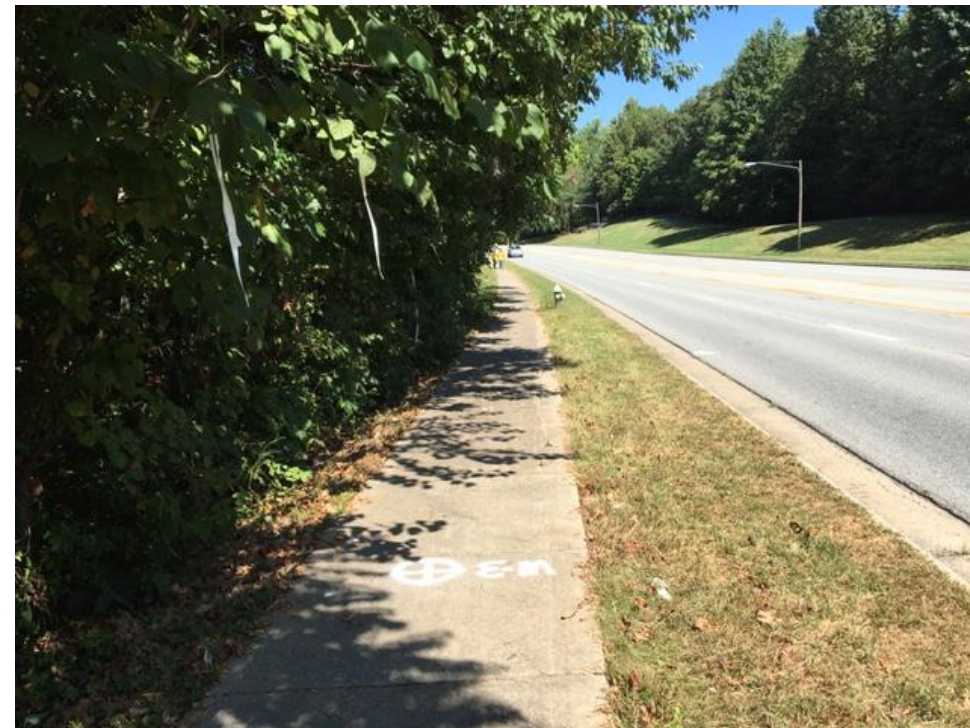
Photograph No. 4: Left of the I-85 Bypass -L- alignment, looking North along proposed End Bent No. 2.
