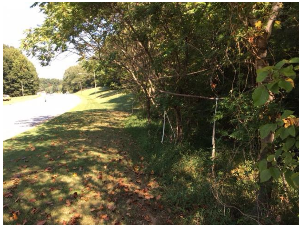
Photograph No. 2: Left of the I-85 Bypass -L- alignment, looking North along the proposed End Bent No. 1
