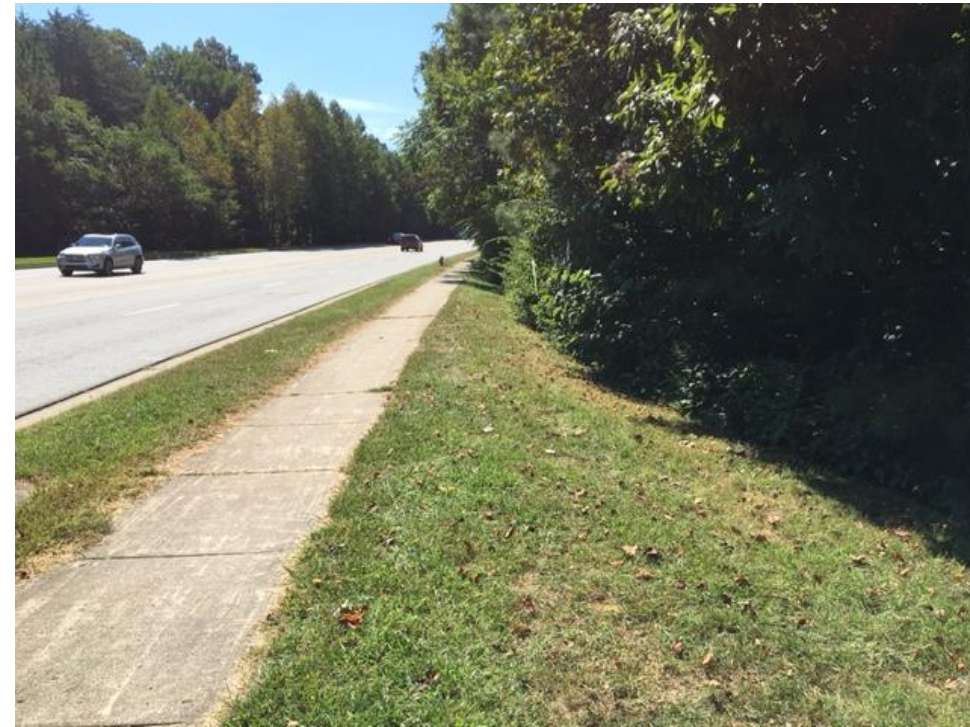
Photograph No. 3: Right of the I-85 Bypass -L- alignment, looking South along proposed End Bent No. 2.
