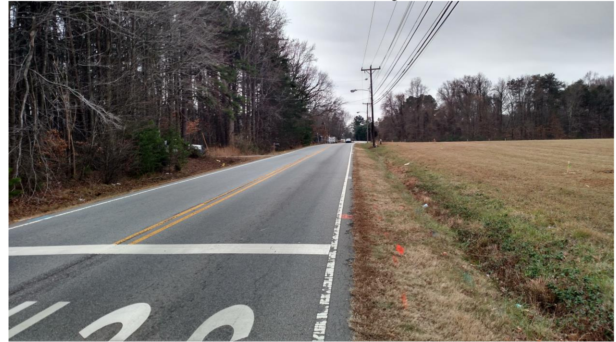
View Looking Downstation Along -Y5-
