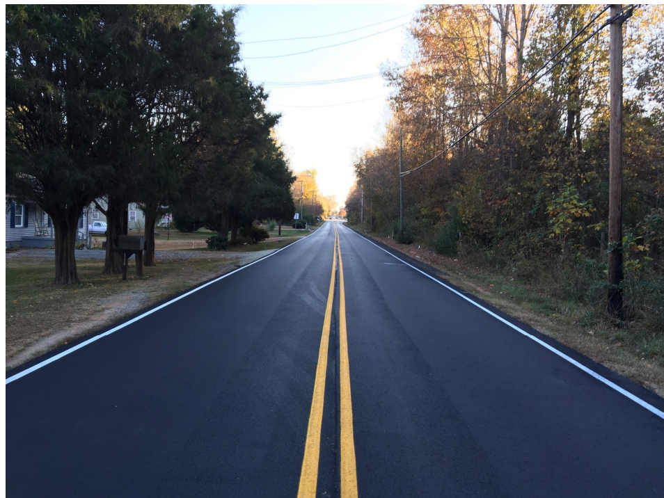
Photograph No. 2: North Approach to End Bent No. 2 on Yanceyville Road (-Y4-), looking South.
