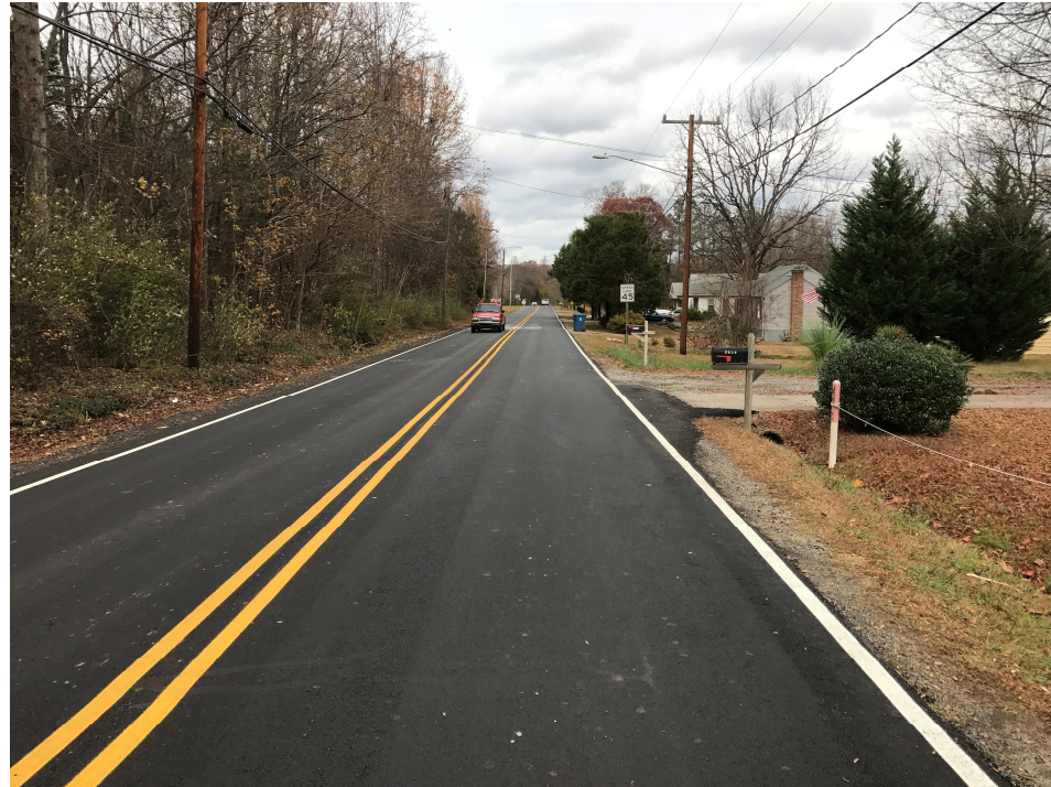
Photograph No. 1: South Approach to End Bent No.1 on Yanceyville Road (-Y4-), looking North.
