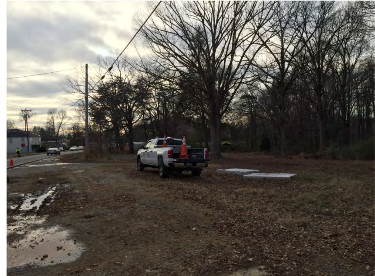
PHOTOGRAPH 2: VIEW OF -Y16- LOOKING SOUTH FROM NEAR CENTER OF PROPOSED BRIDGE.
